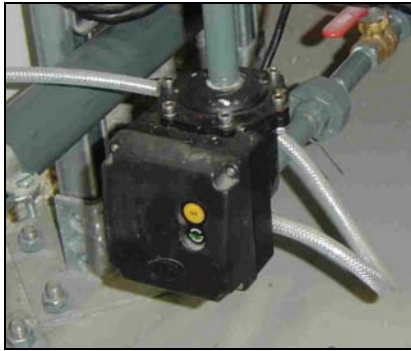
Figure 14 - Example of Zero Air Loss Drain
