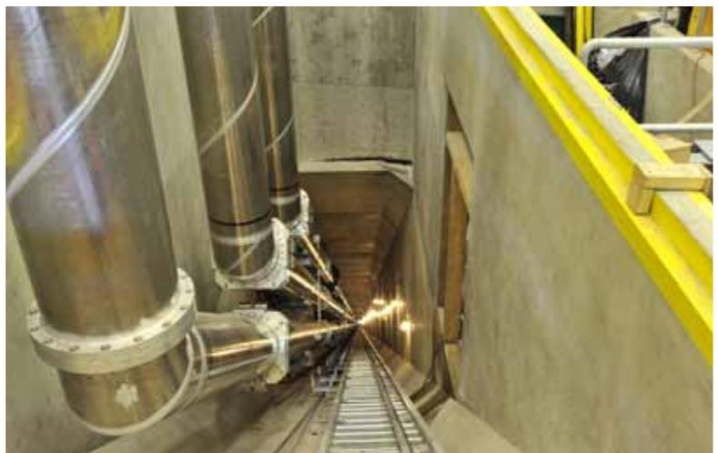
Gas-insulated conductors installed in Mica leadshaft.
