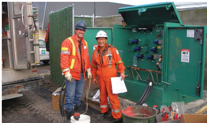
Roger Lamothe, trades trainee, (left) and Goan Yim, power line technician, (right) working on the electrical terminations to energize a padmount transformer servicing the broadcast tent at the Vancouver Olympic Centre Hillcrest curling rink.
