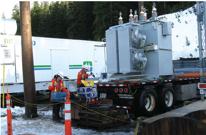
Matthew Betts, power electrical equipment technologist and Debie Ocampo, engineer in training, commissioning one of the Cypress Mountain diesel generation station transformers that was on standby as emergency back up power during the Games.
