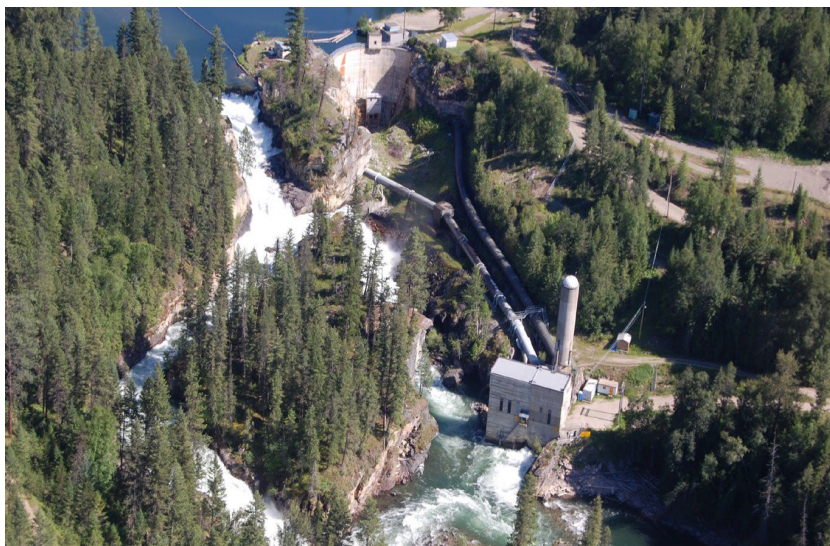
Wilsey Dam and Shuswap Falls generating station
