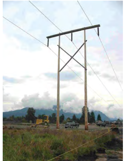
Example of an H-frame structure
