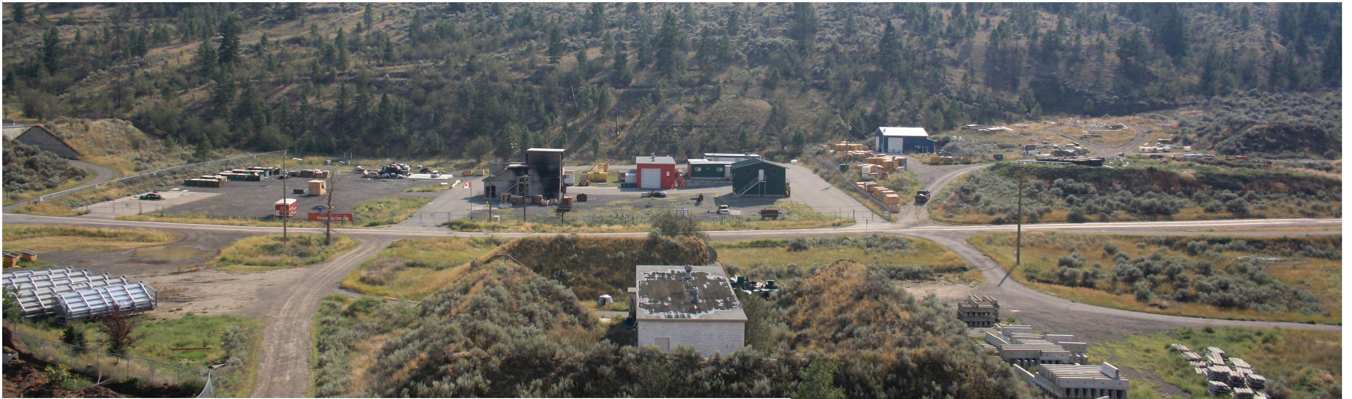
Existing view of City Works Yard property for substation looking towards Kenna Cartwright Park
