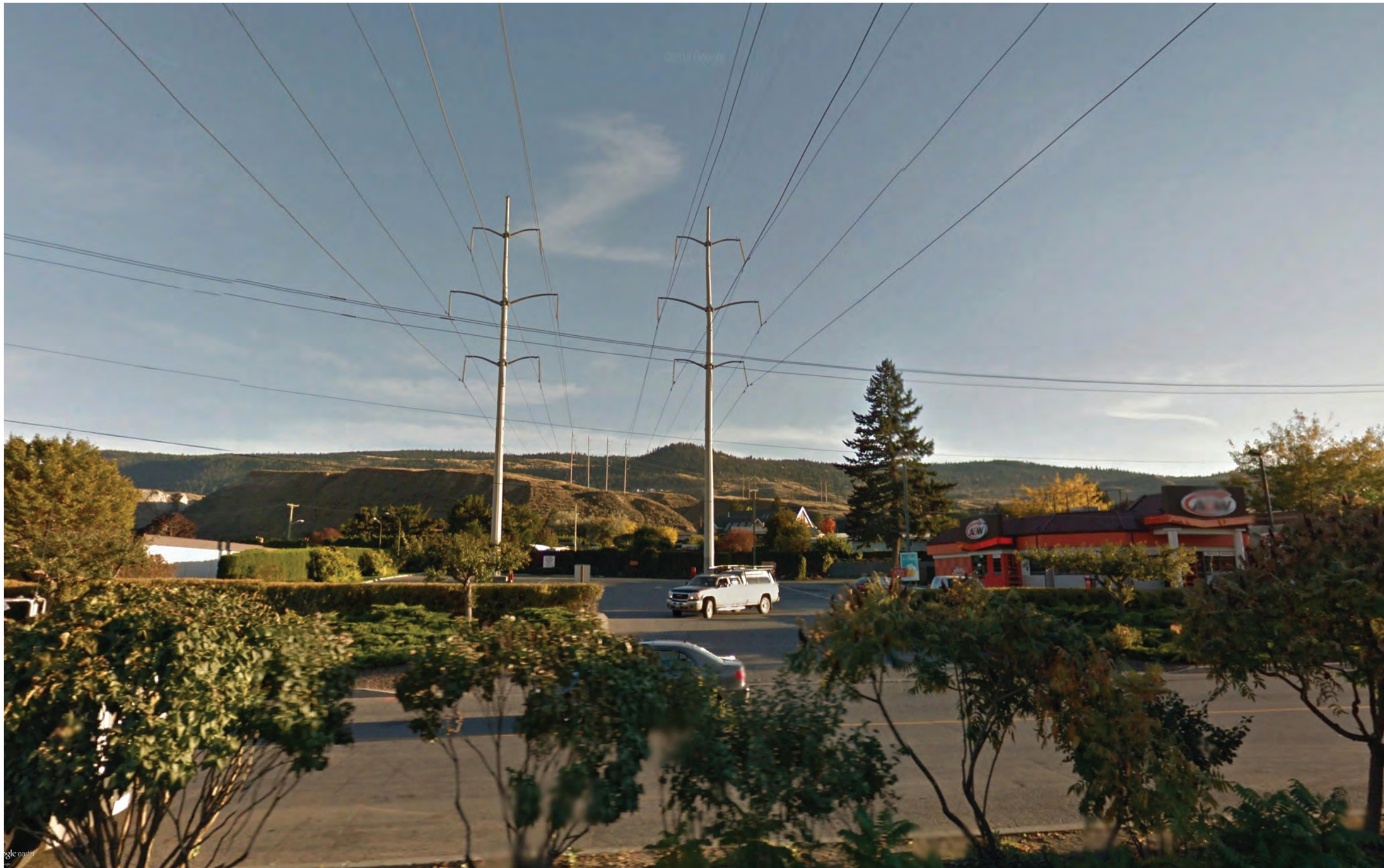
Example of poles to be used in Kenna Cartwright Park
