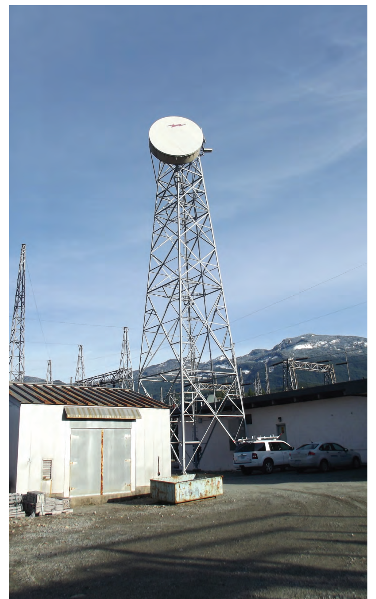
Similar 24m tower with one microwave dish (3.6m in diameter)
