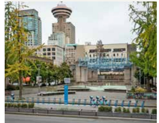
Underground substation at Cathedral Square Park, Vancouver
