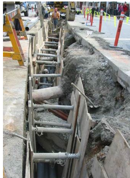
Constructing an underground duct bank, and crossing other utilities, in downtown Vancouver
