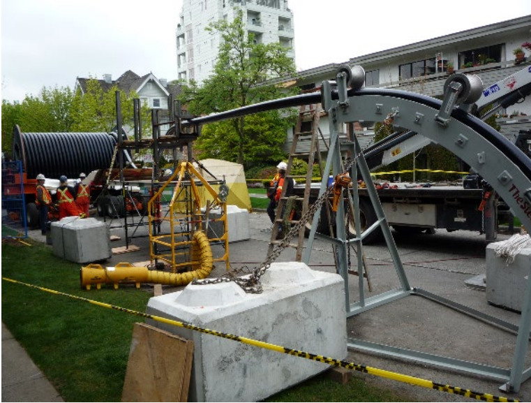
Example of pulling cable into underground vault and duct bank
