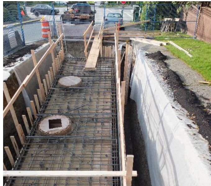
Vault form in Metro Vancouver
