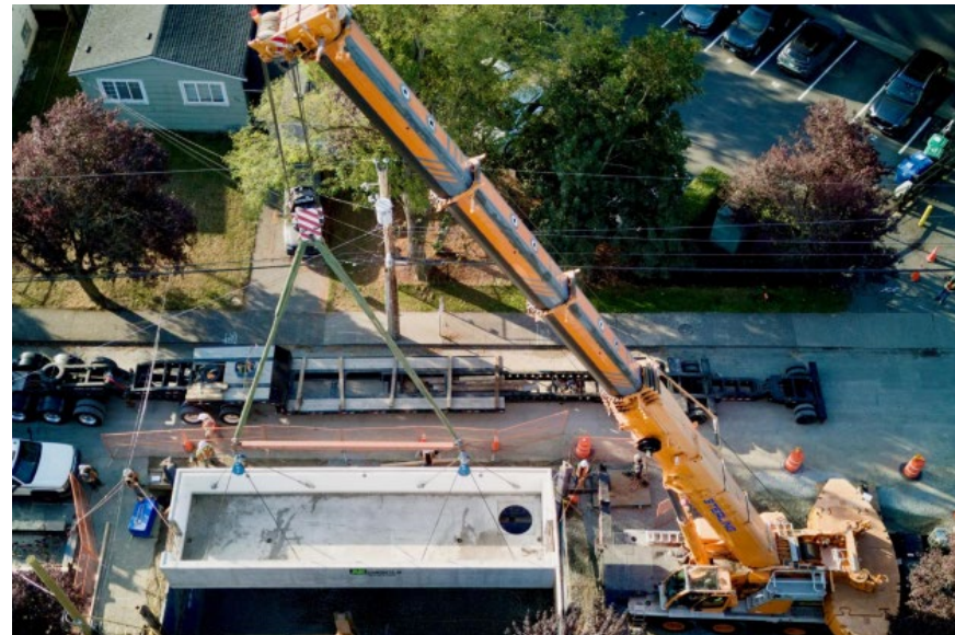
Pre-fabricated vault installation in Victoria, BC
