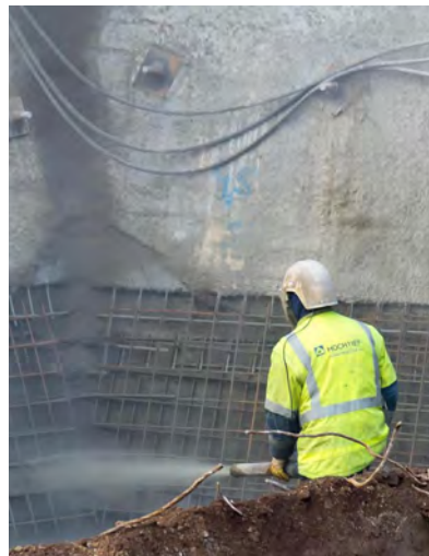
Example of shotcrete application to stabilize an excavation
