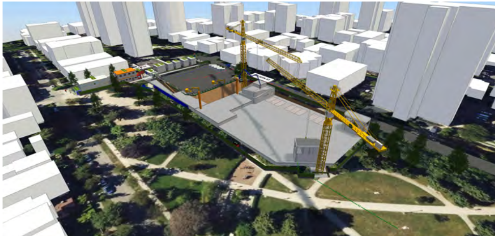
The roof of the substation is in place and work is taking place out-of-sight
