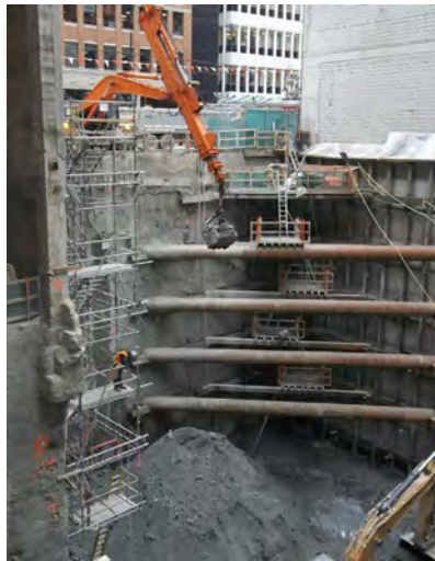
Example excavation in downtown Vancouver
