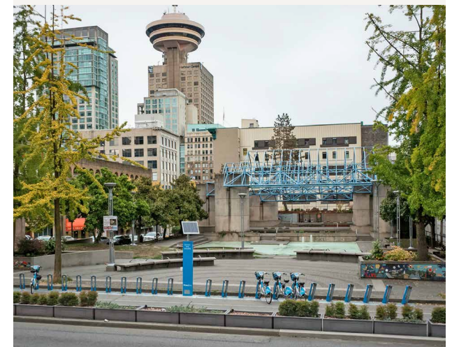
Underground substation at Cathedral Square Park, Vancouver
