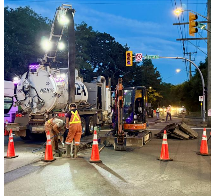
August 26: Investigate work taking place at night at the Interurban Road and Wilkinson Road intersection.
