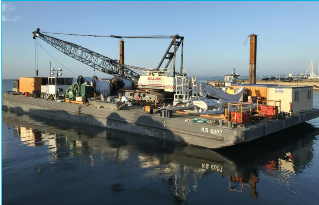
Photo example of barge and power line cable work.
