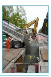
Place in concrete, wait for it to set, then remove the form.
