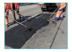
Refill the trench and repair the roadway.
