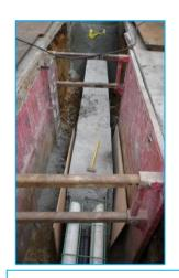
Create a form to hold the concrete in the right shape while it sets and add PVC ducts that will hold the cables.
