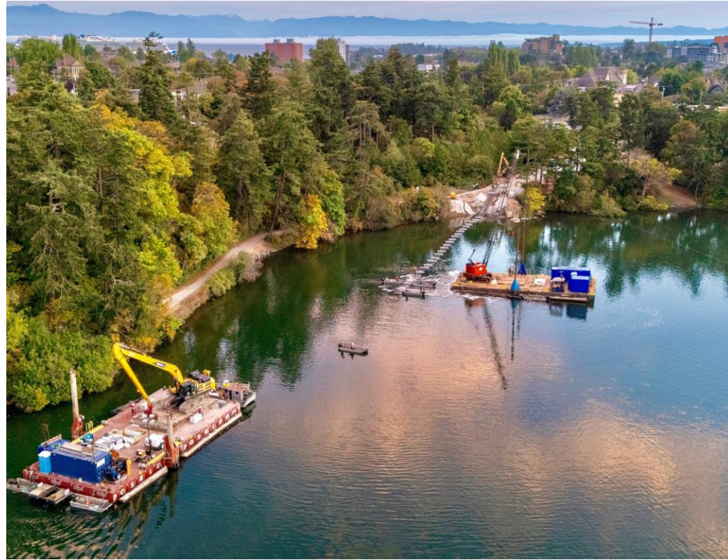
August 21: Evening view of the successful sinking of the conduits into the marine trench. Only five days of the possible ten-day marine navigation closure was required.
