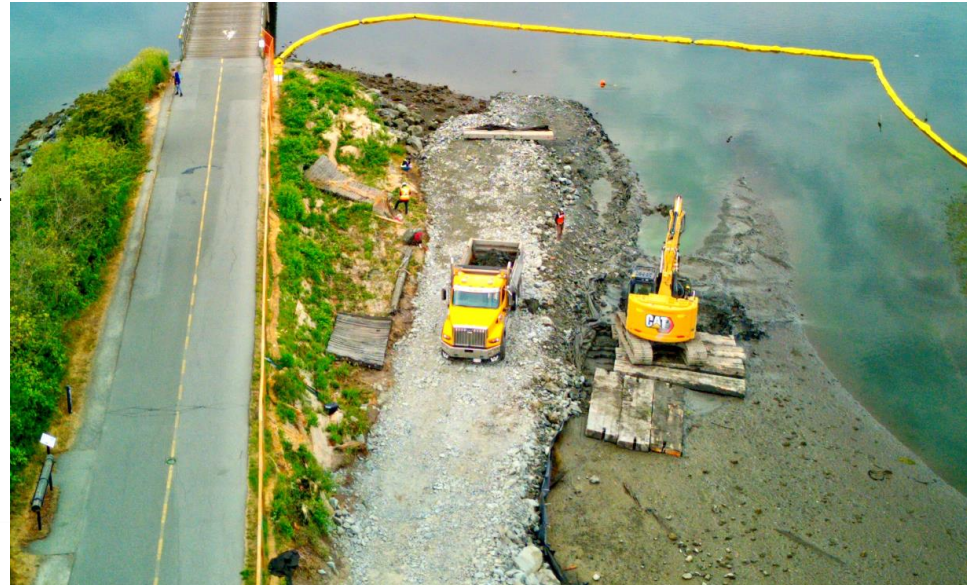
July 16: Trench work within the Viaduct Park foreshore area.
