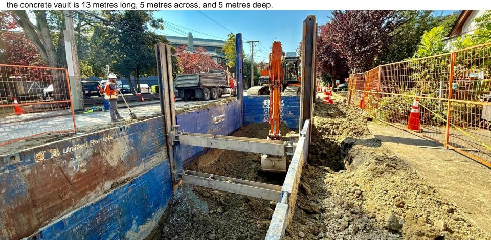
September 16: The completed excavation for the concrete vault placement. The lower section of the concrete vault is on the left.
