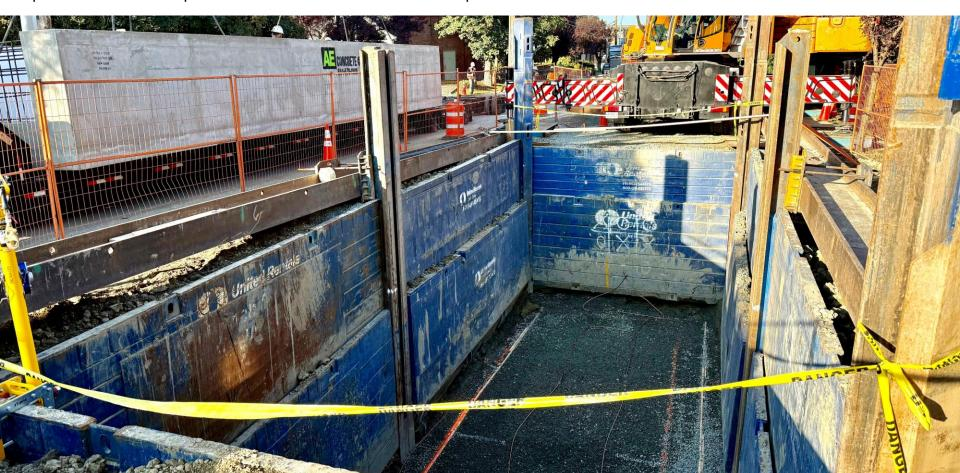
September 16: Crews making final checks to ensure a safe and secure lift of the lower section of the concrete vault. The first concrete vault for the project was successfully placed on Dunedin Street.
