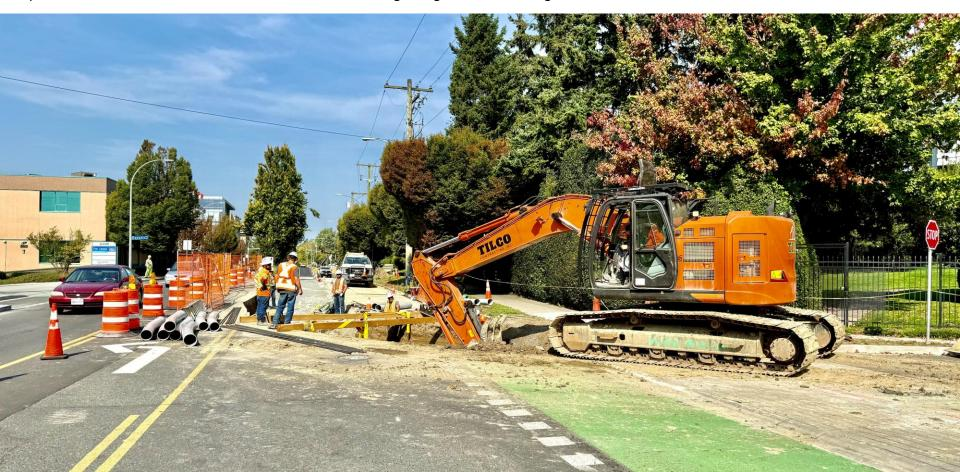
September 3: Placing curving duct bank along the trench as we turn off Gorge Road and onto Dunedin Street.
