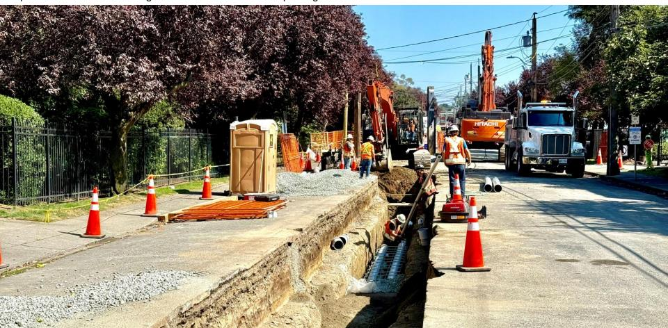
September 11: Excavating material for the duct bank, and in the background, placing a section of sheet pile for the concrete vault
