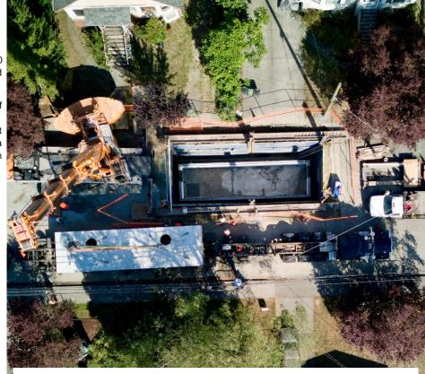
A September 16 bird's-eye view of the concrete vault placement on Dunedin Street, with the lower section of the concrete vault in place and the top section ready to be lifted into place.
