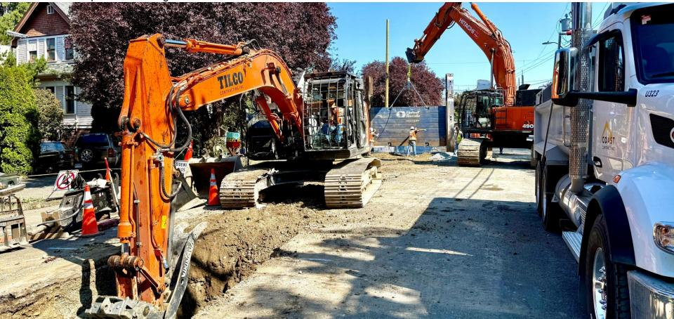
September 11: A broader view, looking westward, of the sheet pile shoring in place and the removal of material. The excavation for
