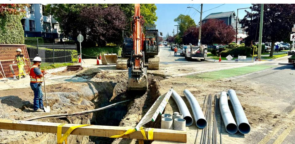
September 11: Crews moving down Dunedin Street and placing the duct bank conduit.
