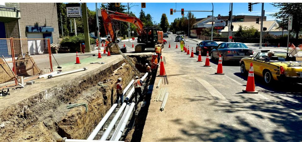
August 7: Crews connecting a section of conduit together. The conduit ends are glued and then knocked in to have one cohesive pipe.
