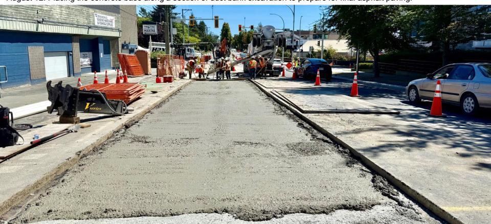
August 15: View westward down Gorge Road showing duct bank work at an intersection with many utilities to work around. Planned
