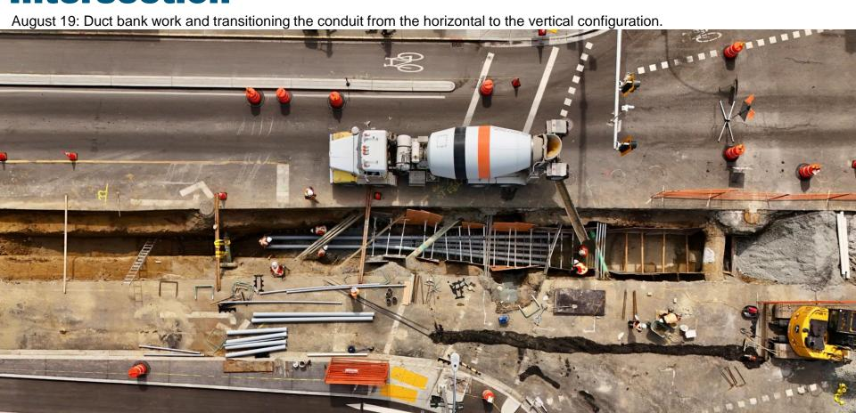
August 19: Placing the conduit and in the background, placing concrete over a section of completed conduit. The trench depth reached just over 3 metres allowing the conduit to be placed under other utilities in the street.
