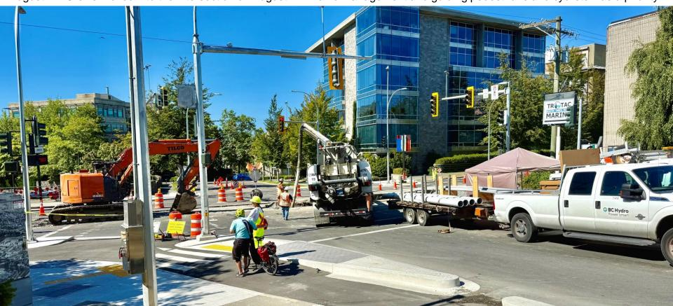
August 12: Duct bank work with soil removal and the excavation work around various underground utilities.
