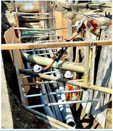
August 19: The complexities of placing the transmission cable duct bank around other utilities and keeping crews safe by placing shoring on the sides of the trench.
