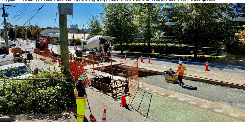
August 7: A closer view of the duct bank work and the placement of a special thermal concrete to keep the cables cool when at or below a 2.5 metre depth.
