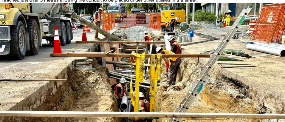
August 19: Conduit placement work, and in the foreground, and the narrowing of the trench width and slowly rising to a 2-metre depth.
