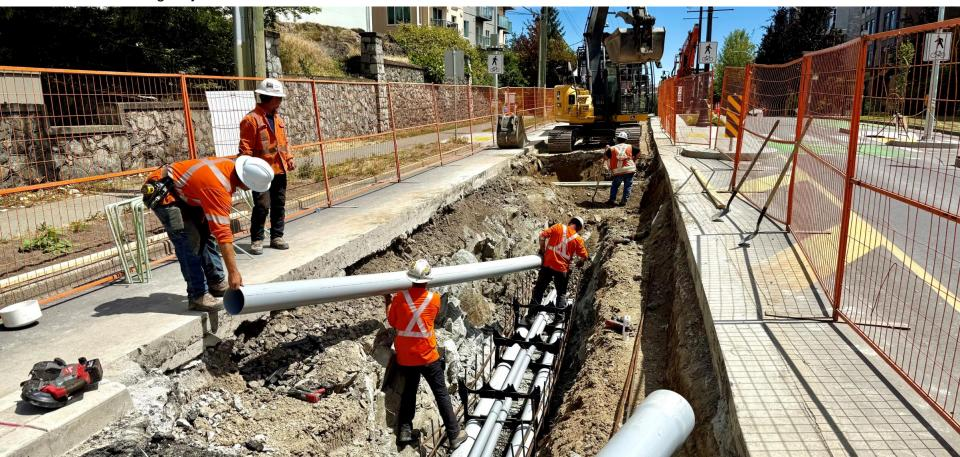
July 8: In the background, concrete is placed along the conduit. In the foreground, material continues to be removed to progress down Gorge Road. The three red lines on the road show the location of the streetlight electric conduit and the careful excavation around them.
