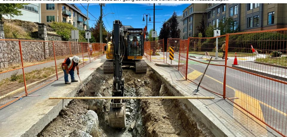
July 8: With a section clear to begin the placement of the conduit, crews place the spacers and rebar.
