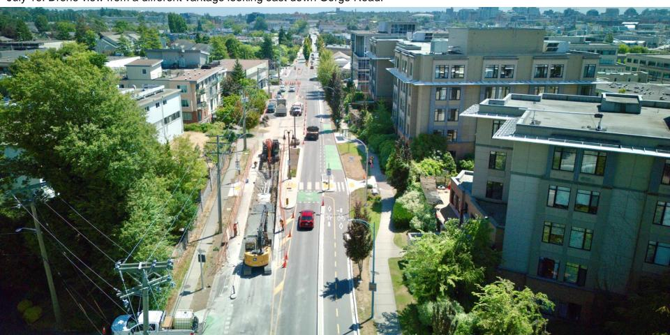
July 23: Placement of concrete over the conduit. The duct bank excavation work finally moved out of the bedrock on July 23 with the trench work now moving through Victoria clay.
