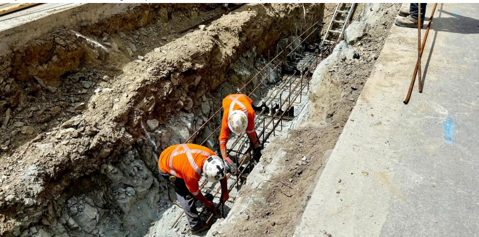
July 8: With the first row of spacers and rebar in place, crews place the conduit.
