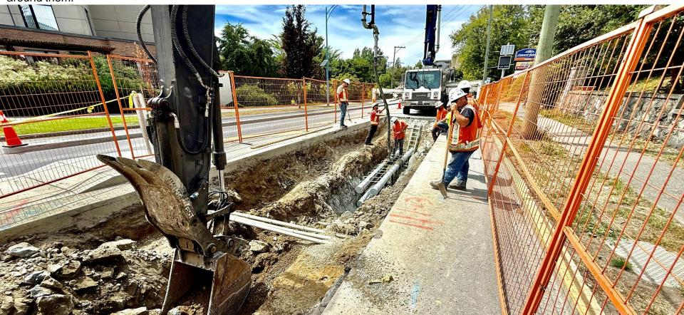
July 16: Electrical caution tape is placed above the duct bank to prevent future excavation in the same location.
