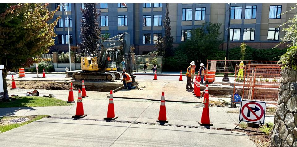
July 23 (evening): Daylighting work to determine underground utilities at the Jutland Road intersection. This investigative work helps to limit any potential delays when the duct bank is built through the intersection in mid-August.
