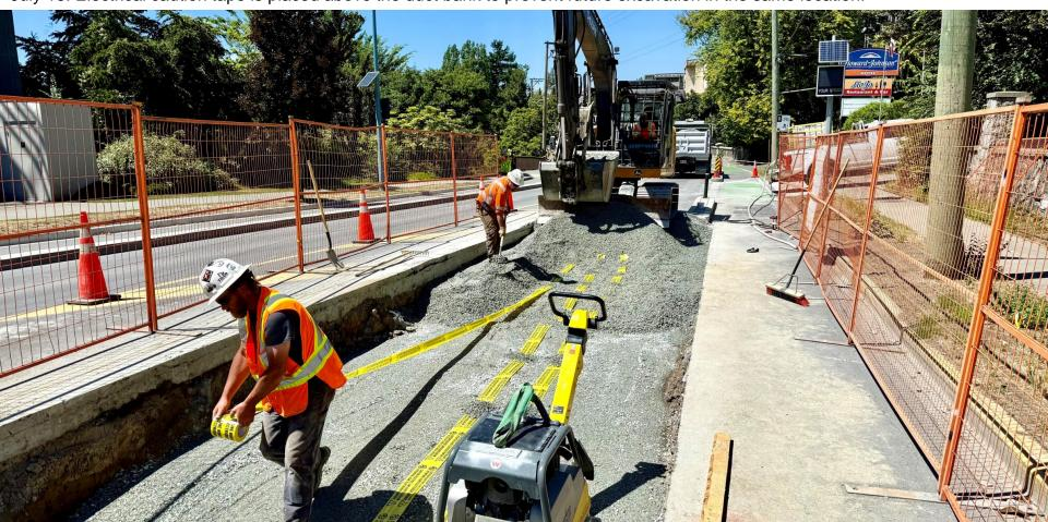
July 16: Removing loose rock from the trench while protecting an irrigation line. The pipe to the left of the excavator bucket is an abandoned water main.
