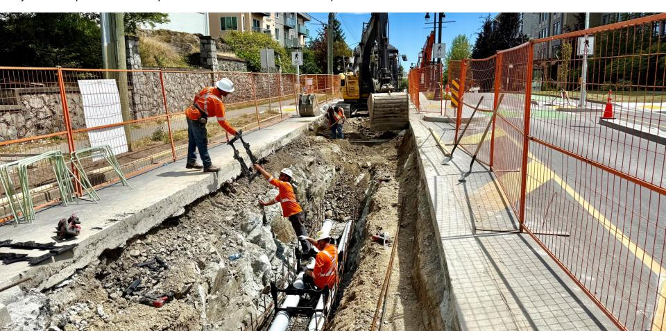
July 8: The second level of conduit placement. There are four conduits that will house the cable, with one conduit used as a spare in the event of an emergency.
