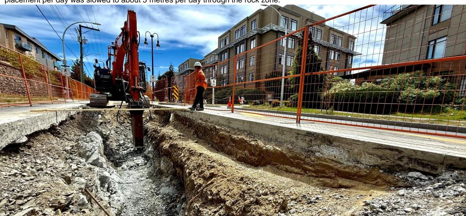
July 8: A second excavator was used to remove the chipped rock material from the trench into a dump truck. The excavators switched positions multiple times per day. The wood 2x4 going across the trench is used to measure depth.
