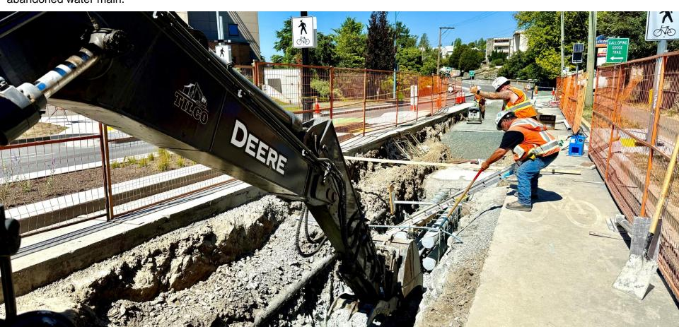
July 16: Rock removal along the duct bank route and confirming the 2.5-metre depth.
