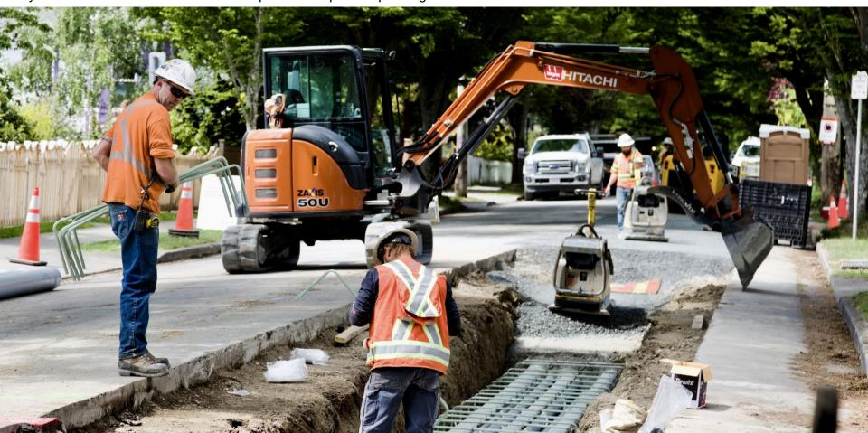
May 21: Compacting fill material above the duct bank.
