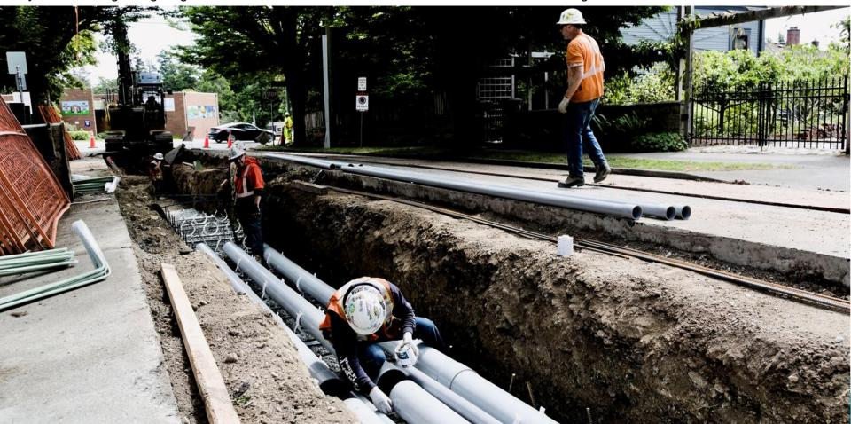
May 21: Duct bank work with the rebar placement prior to pouring concrete.
