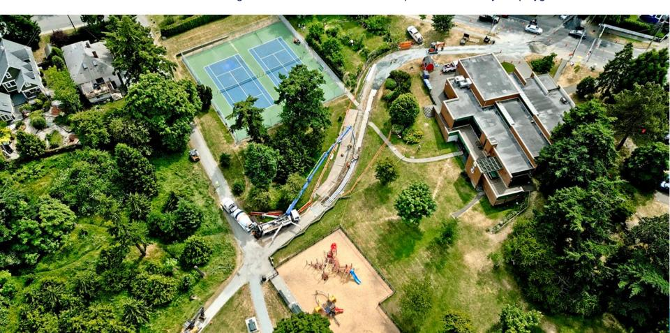
June 11: Another view of the duct bank work and the concrete placement over the conduit.
