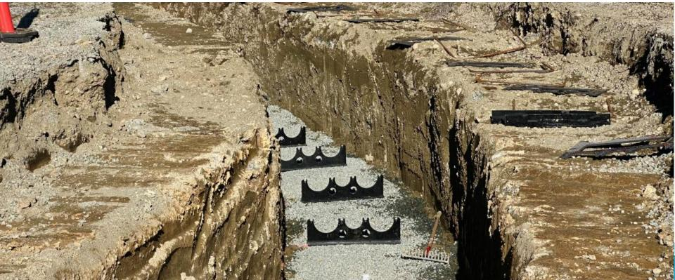
View of the duct bank work with the conduit pipes beginning to be encased in concrete on March 6.
