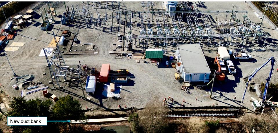
Photo of the duct bank excavation and the placement of spacers to hold the conduit pipe that will contain the cables on March 6. With the work happening within the substation, the excavation was stepped to maintain the integrity of the trench. On city streets, with a narrower work area, and depending on the depth, metal shoring cages may be placed within the trench to maintain worker safety. The soil material is typical Victoria clay.
