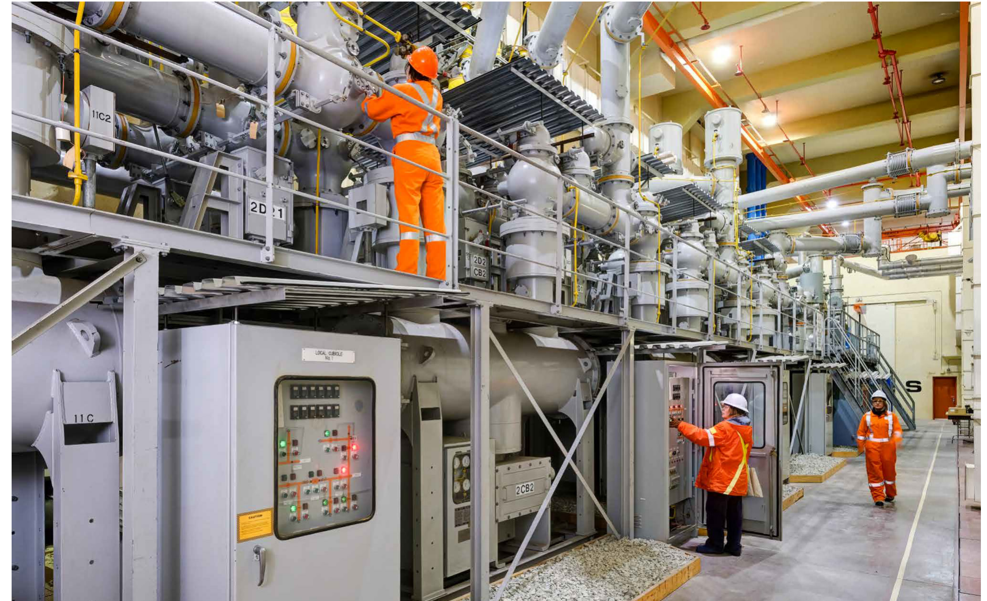
Maintenance at Cathedral Square Substation
