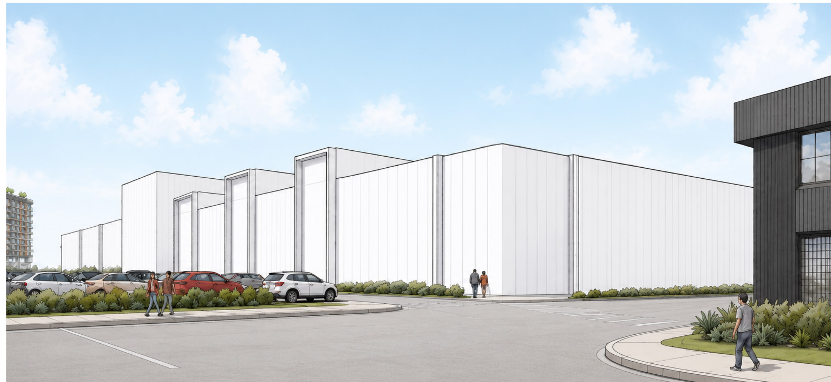
Southeast corner view
