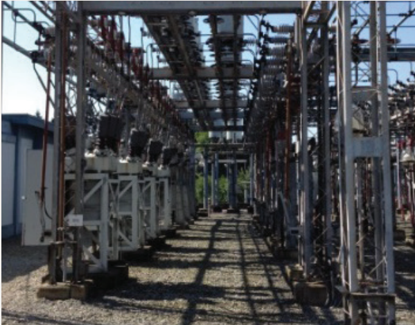
50/60 series outdoor feeder section
