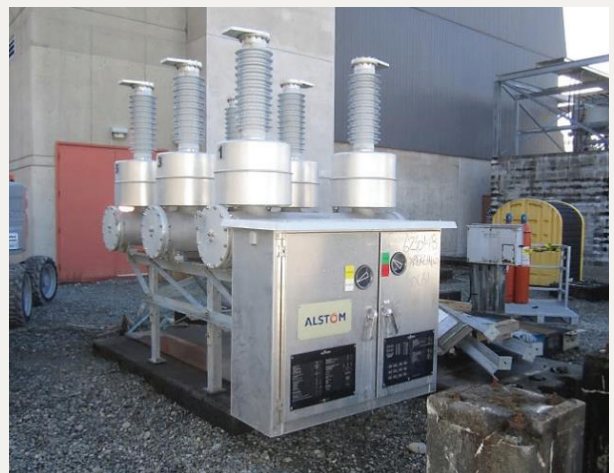
60kV gas-insulated type circuit breaker
