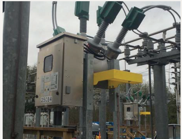
12kV gas-insulated type circuit breaker
