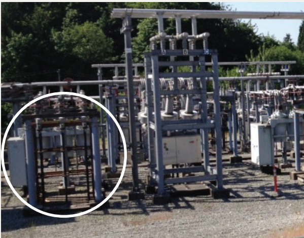
Bulk oil type 12kV circuit breakers
