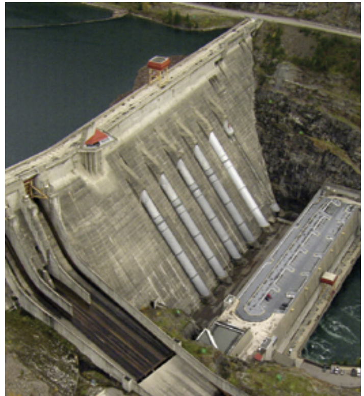
Revelstoke Generating Station
