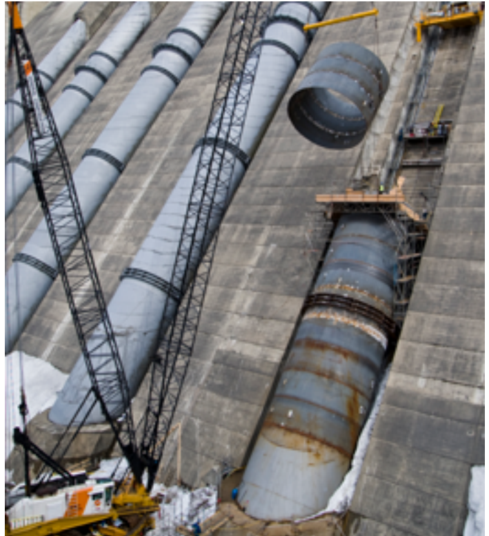
Installing penstock for Revelstoke Unit 5 Project
