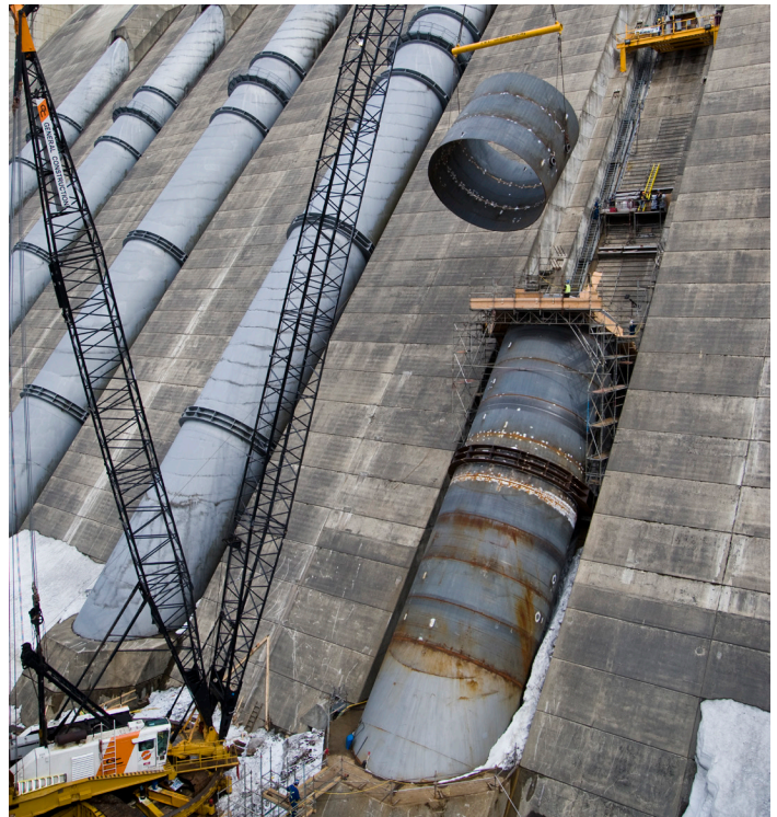
Installing penstock for Revelstoke Unit 5 Project
