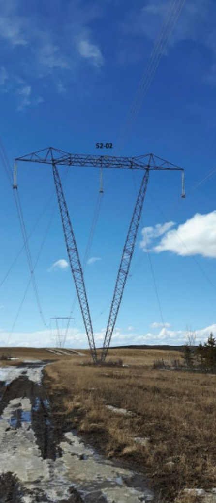
Existing 500kV transmission line
