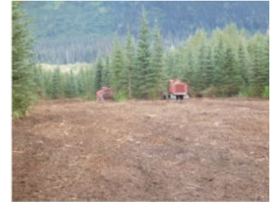
Typical right of way preparation with mulching
