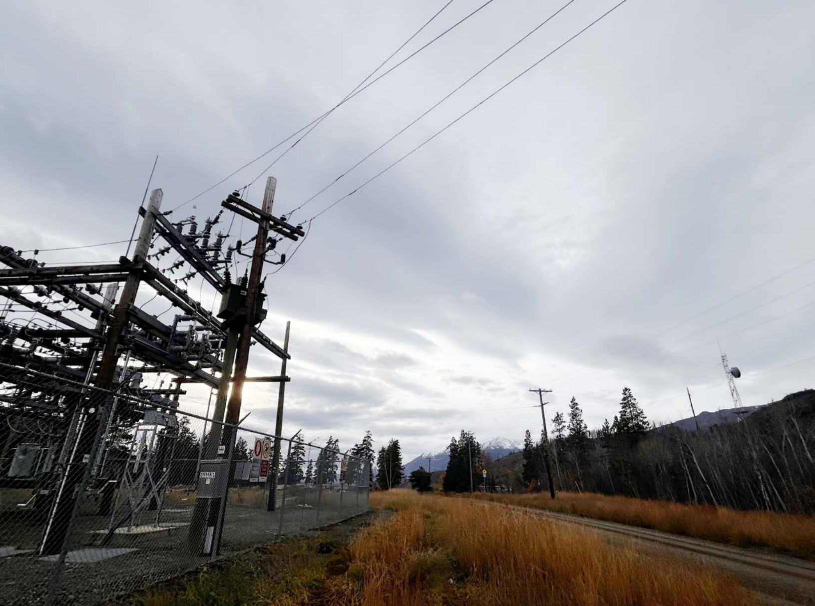
Telegraph Creek. Photo: BC Hydro
