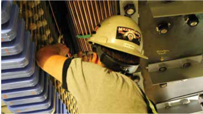
Work on Mica 5 generating unit stator.
