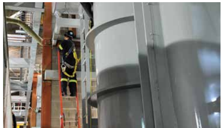
Work on the new switchgear equipment.
