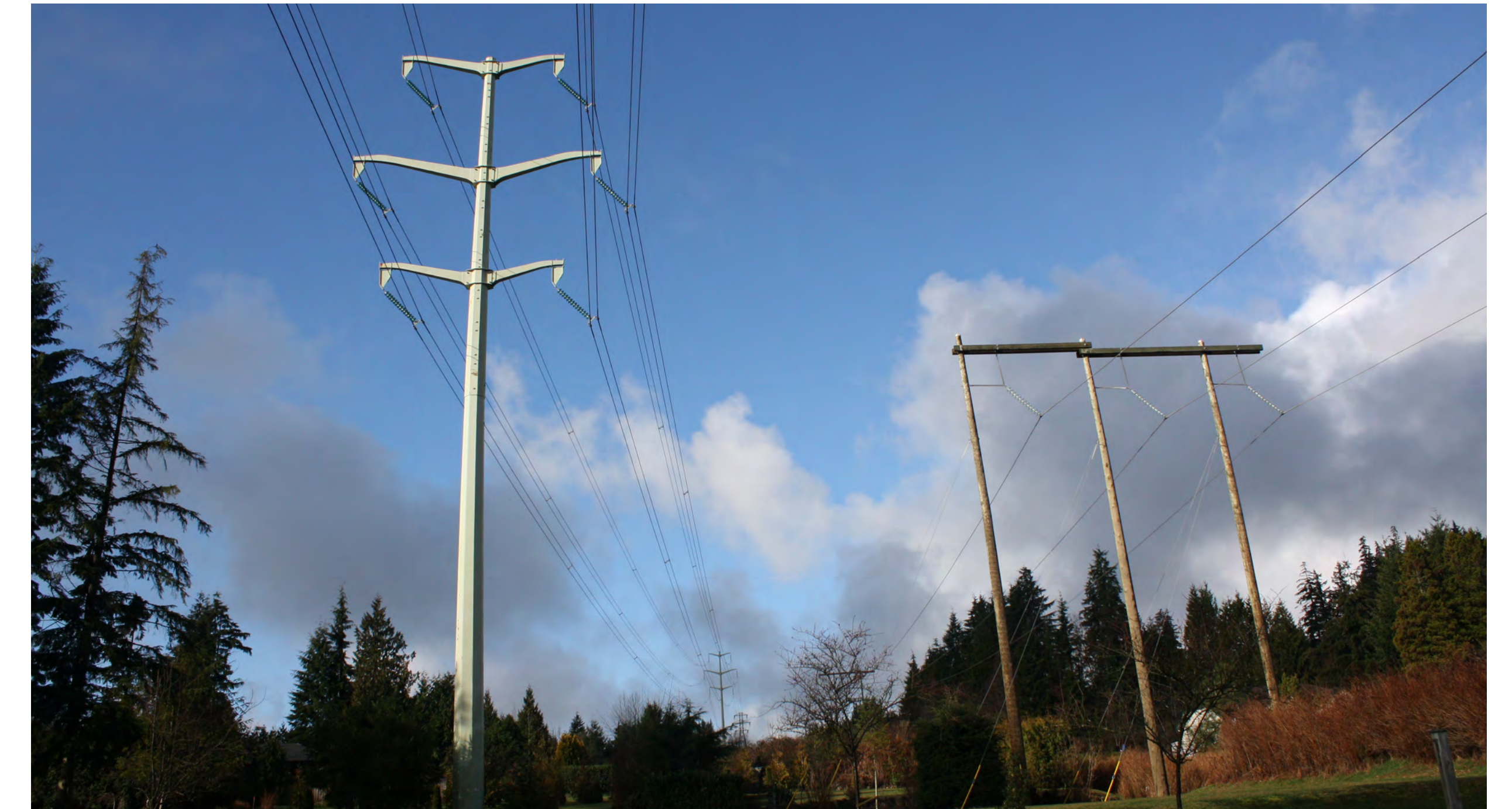
Existing structures (monopole and wooden H-frame) in Anmore
