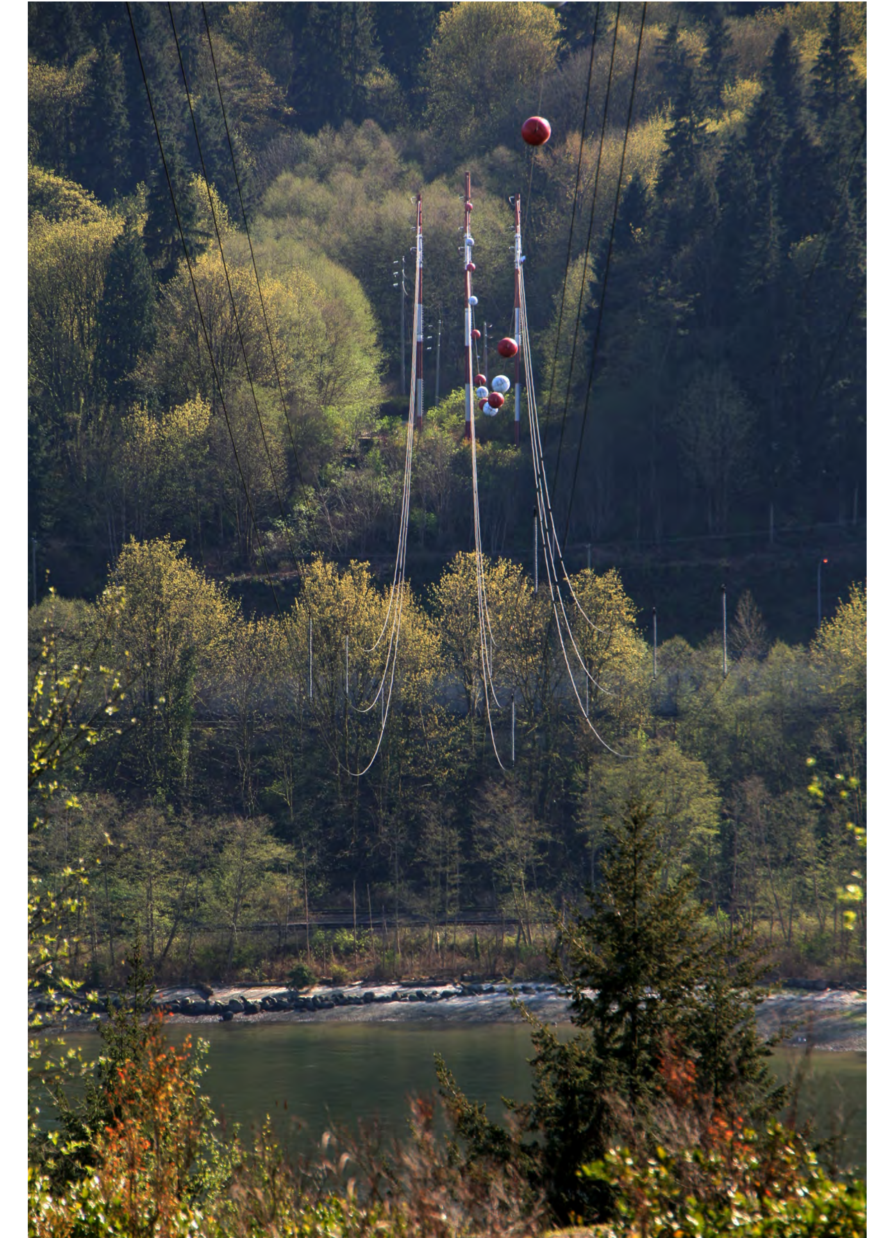
Existing Burrard Inlet crossing, looking south
