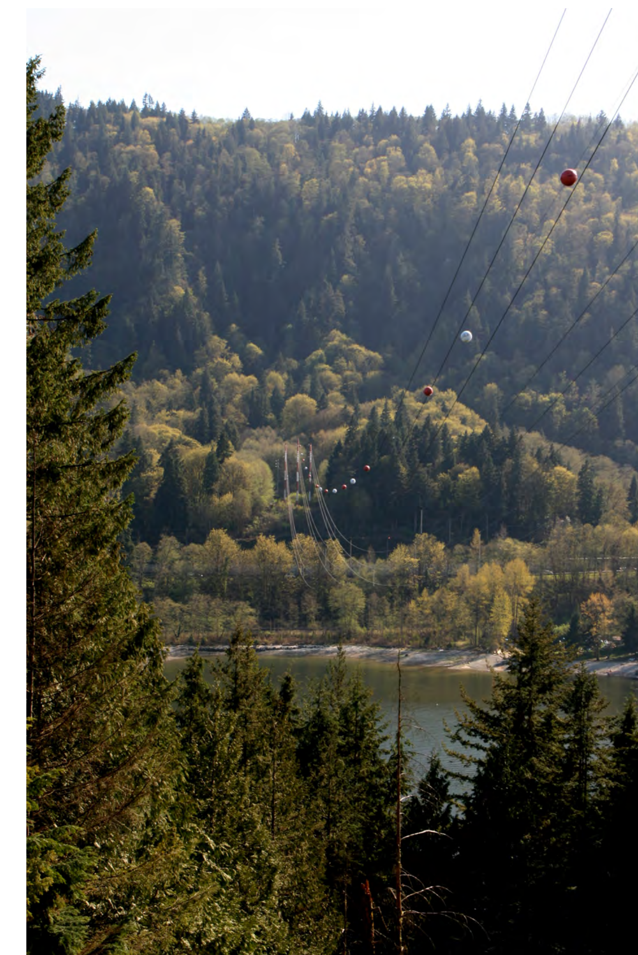
Existing Burrard Inlet crossing, looking south
