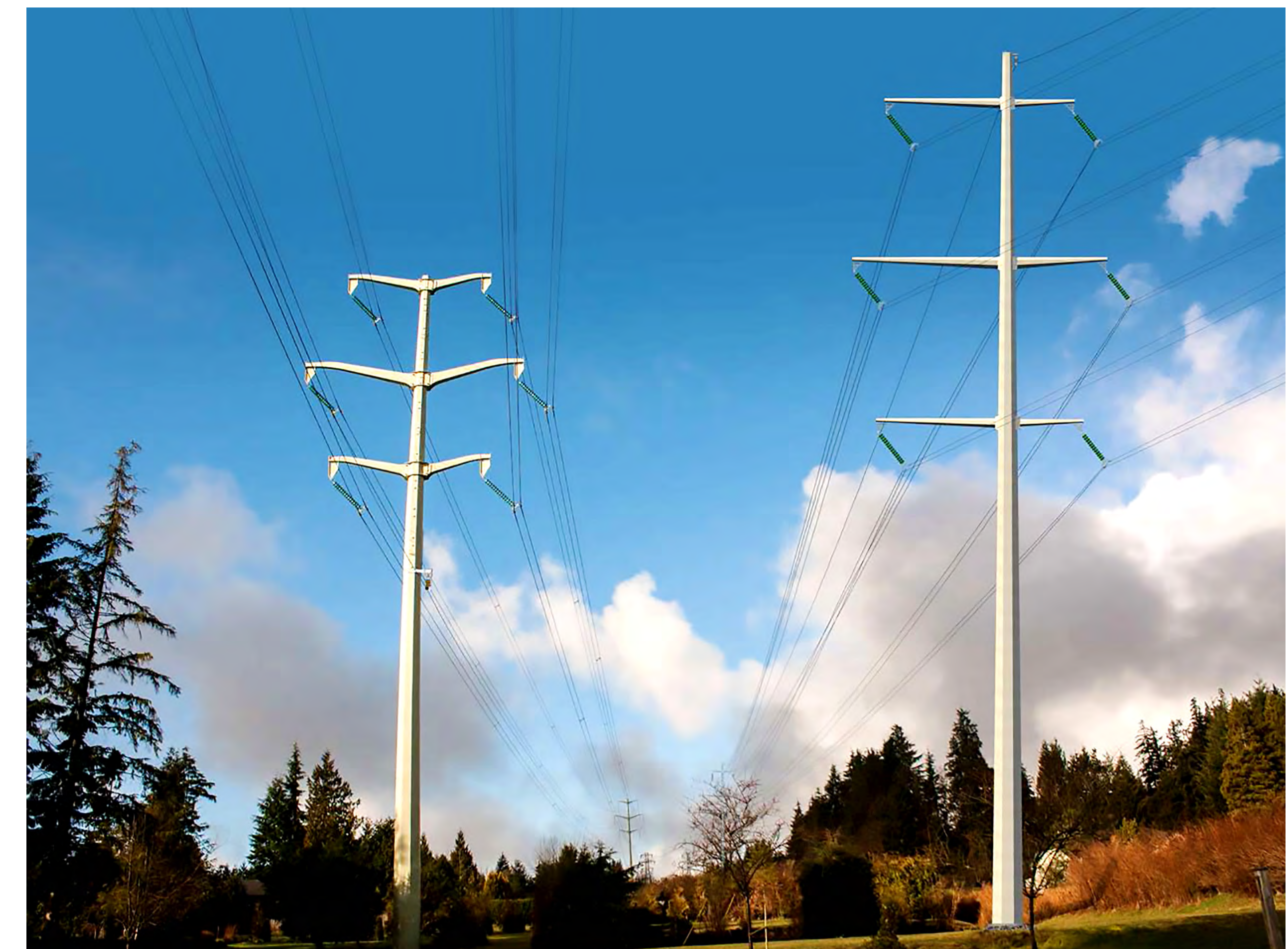
Preliminary rendering showing a new steel monopole replacing a wooden H-frame in Anmore (tower design and placement subject to change). With Alternative 2, there would be 17 fewer poles than existing in the Anmore area.
