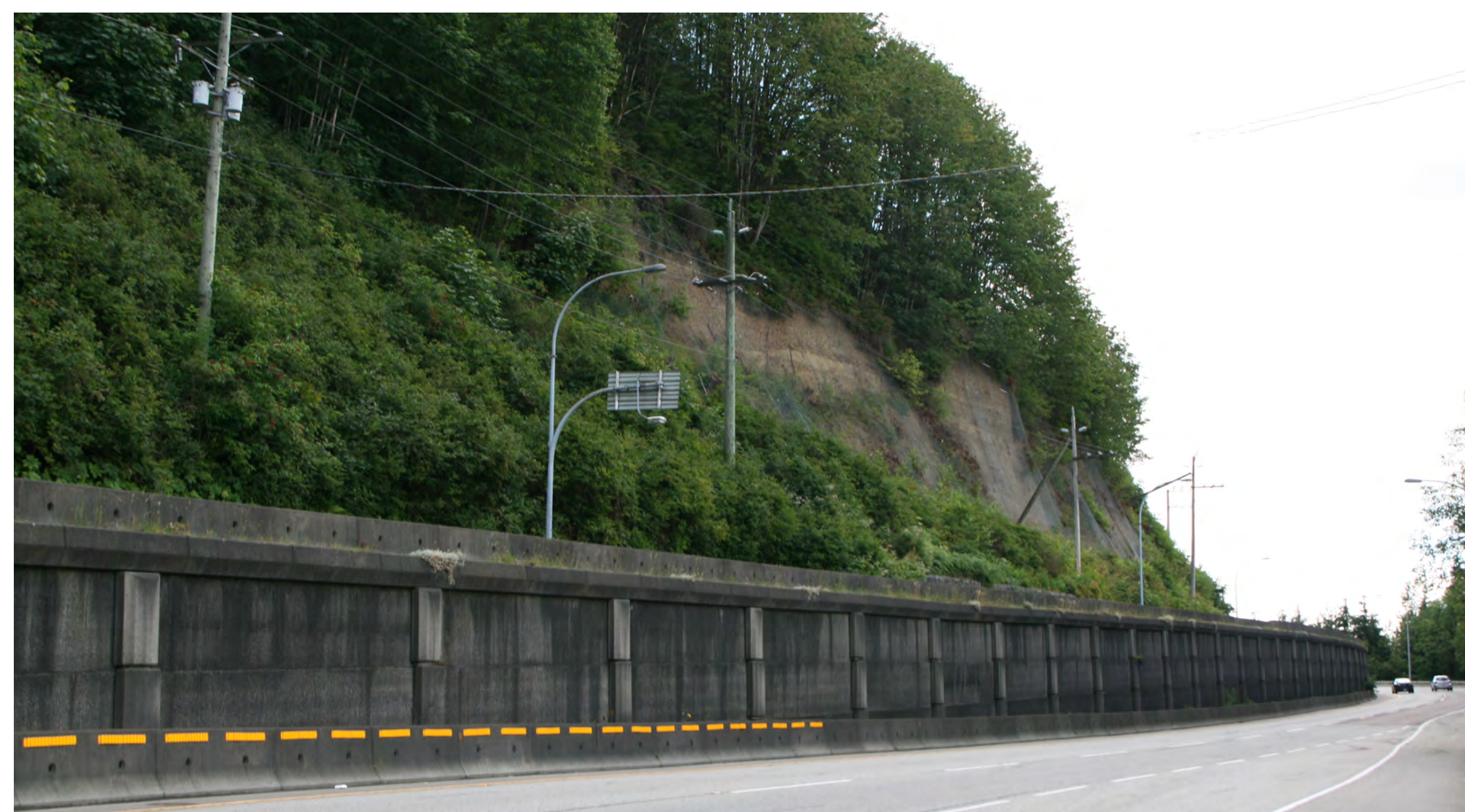
An area of slope instability along Barnet Highway, west of the velodrome
