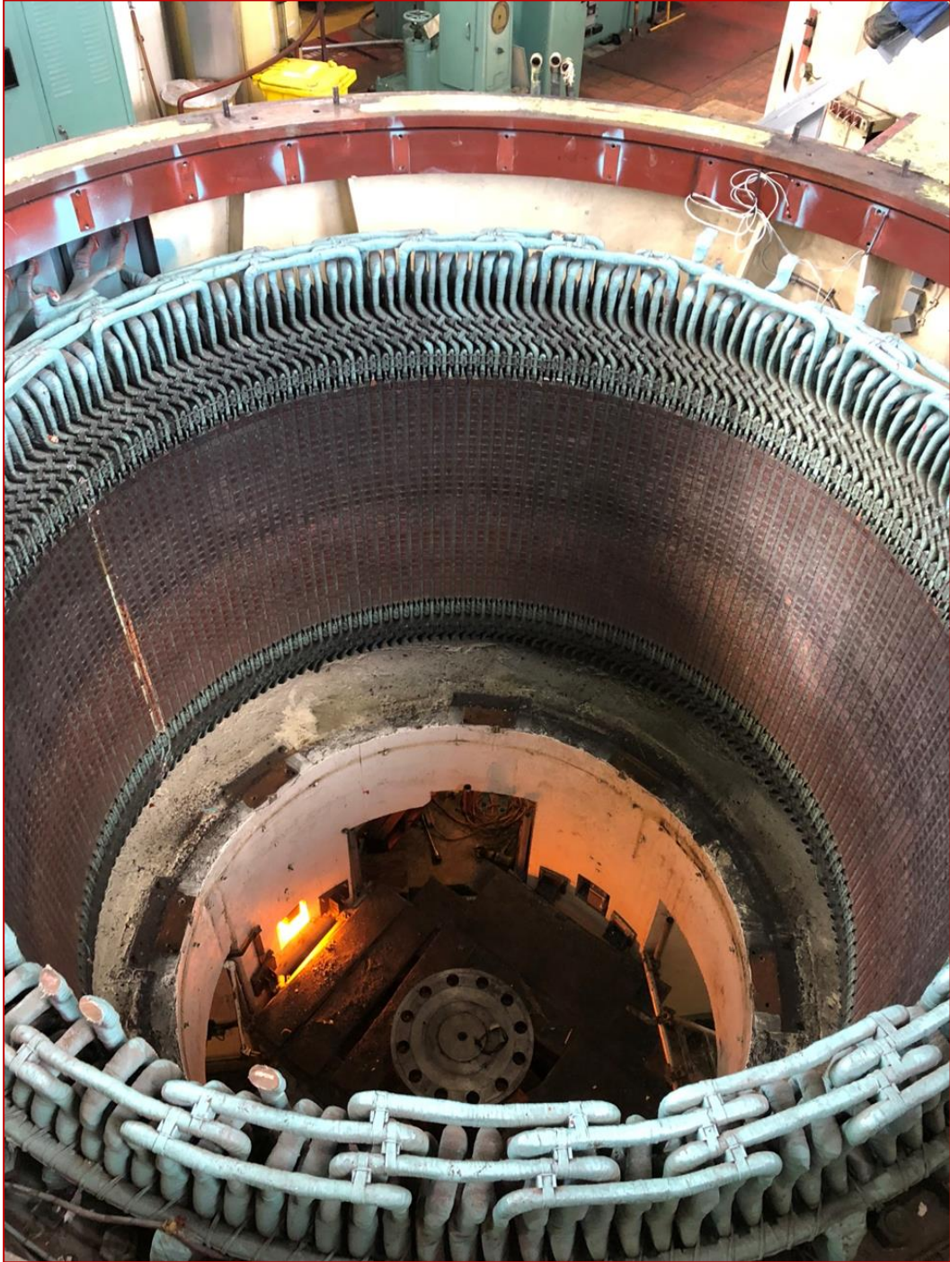
Above, a picture diagram inside the old powerhouse wall of one of the six units. On right, Generators 5 with the rotor and shaft removed.
