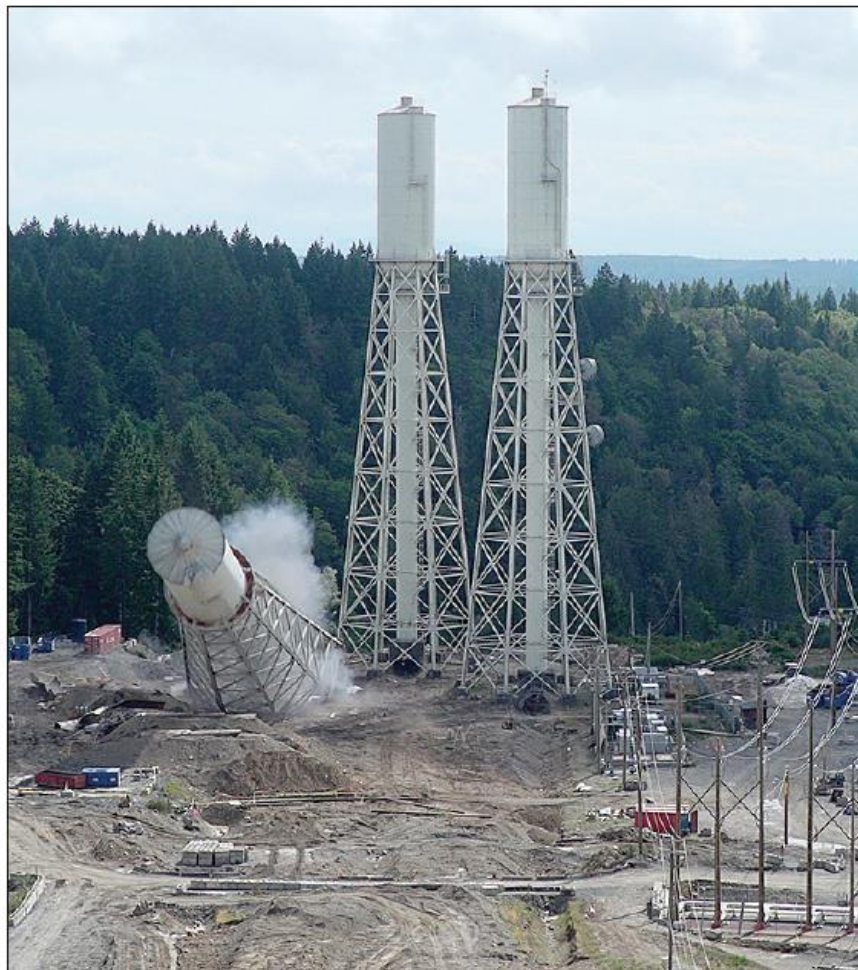
As part of the John Hart decommissioning work, the first of two old surge towers was removed Friday morning. BC Hydro photo
