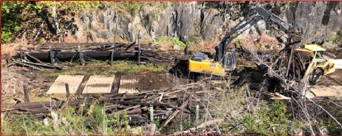
The final piece of woodstave penstock, as shown in the inset photo, was removed on April 30. The general picture is an earlier photo of the near full removal of the penstocks.
