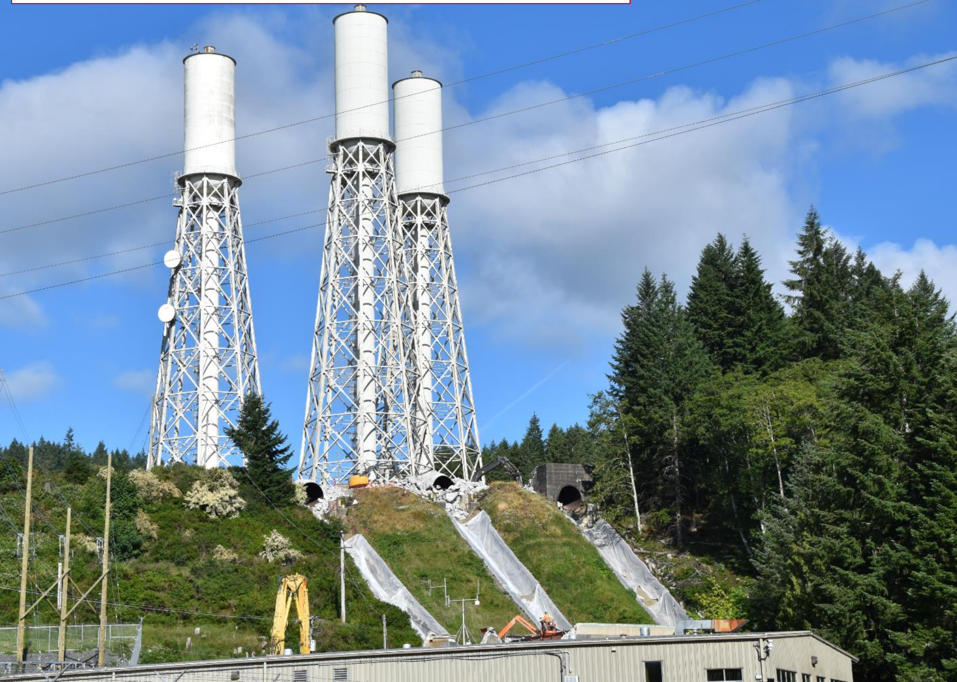
Removal of the anchor blocks and steel penstocks downstream of the surge towers.
