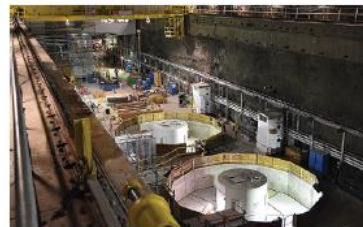
An October photo of the underground John Hart powerhouse. The water bypass facility is located within a lower floor level. BC Hydro photo
