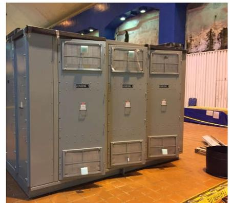
An exciter transformer being installed at GMS.
