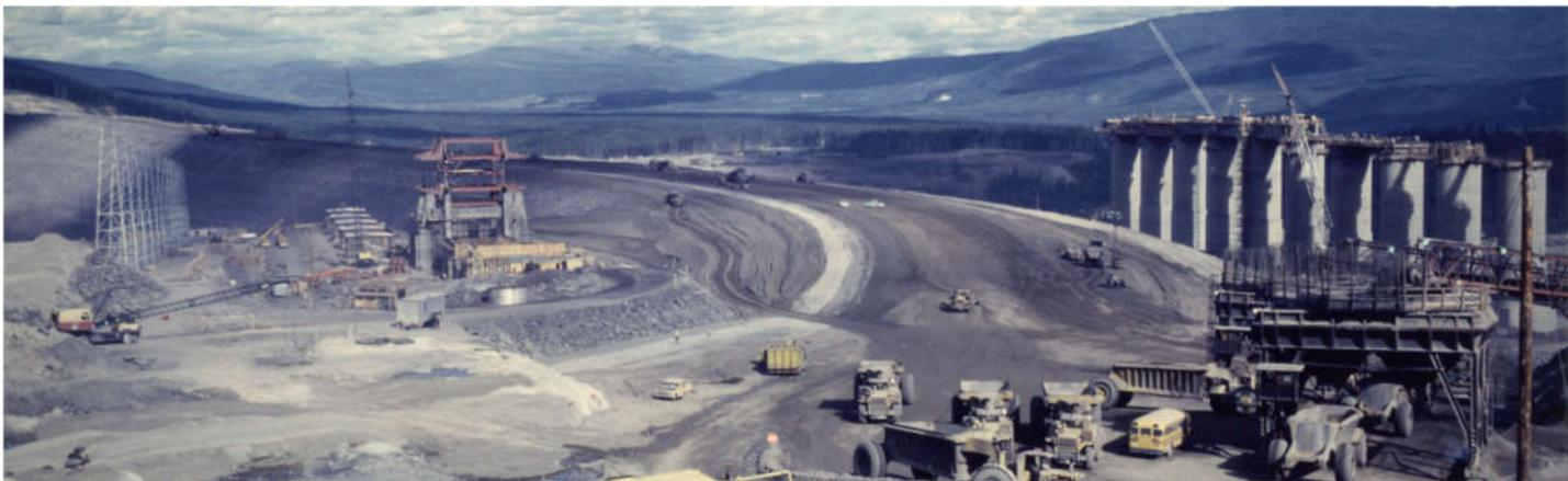
Construction of the intake tower – that passes water through the dam to the generating station - at Gordon M. Shrum (GMS) Generating Station in 1967.
