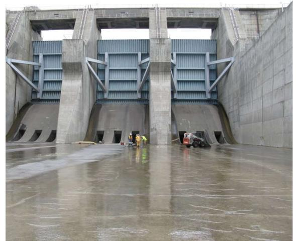
W.A.C. Bennett Dam spillway chute showing the three spillway gates, and the nine sluiceways containing slide gates, from the downstream side.
