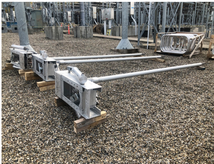
New equipment ready to be installed for the GMS 500 kV Disconnect Switches Replacement Project.
