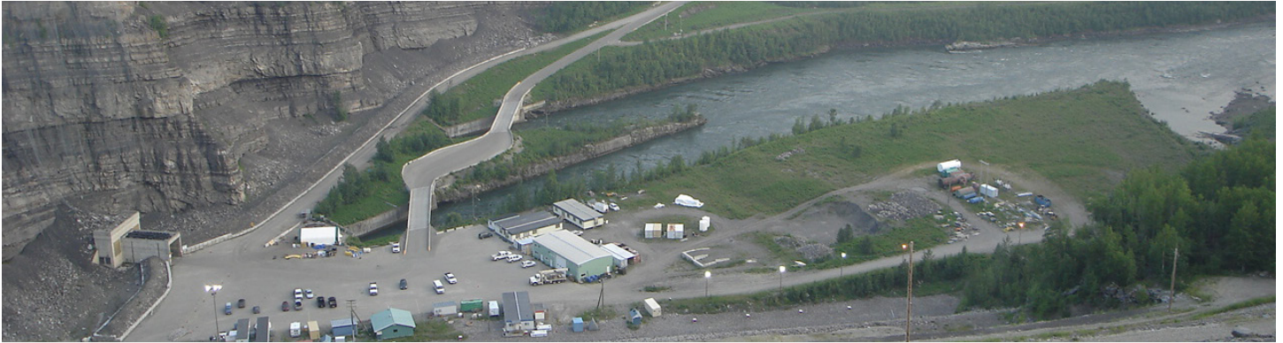
The tailrace – an outlet, downstream of the generating station, which discharges water that has passed through the turbines to generate electricity – at Gordon M. Shrum Generating Station.
