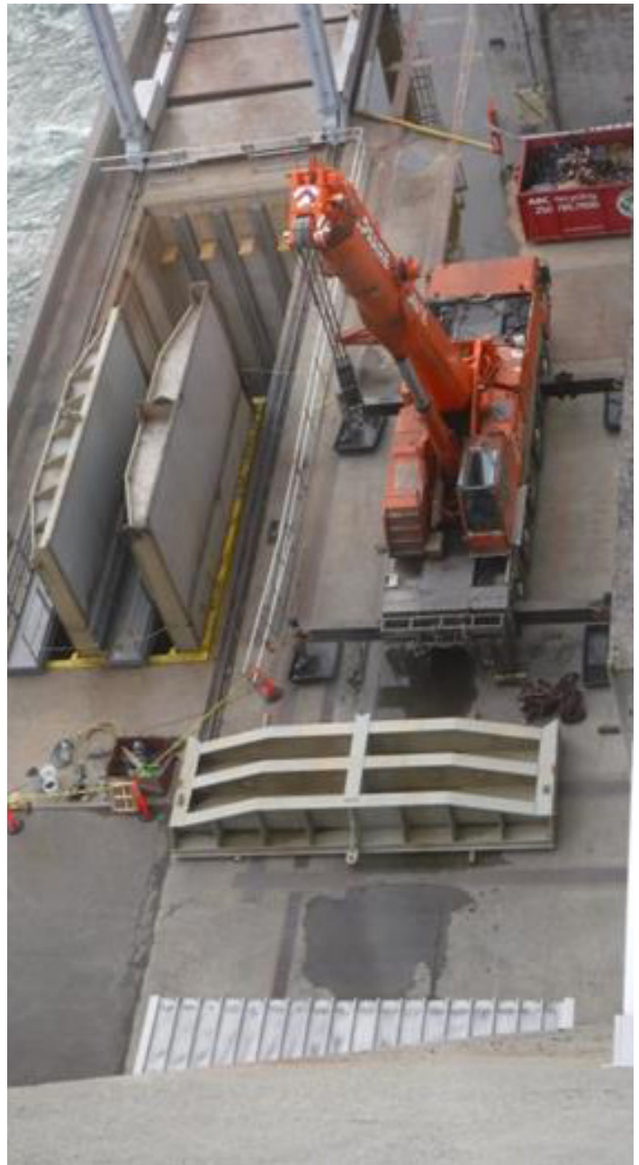
Contractor disassembling draft tube maintenance gates into sections for transport to offsite refurbishment area.
