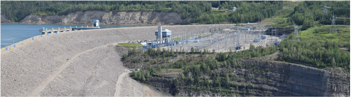
W.A.C. Bennett Dam is an earthfill embankment dam and is 2,040 metres across the top, 183 metres high and 800 metres thick at its base.
