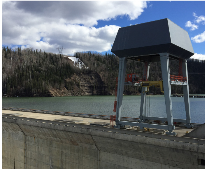
Peace Canyon Dam deck and crane.
