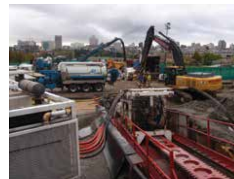
HDD rig and staging area on the Vancouver City Central Transmission (VCCT) Project in David Lam Park, Vancouver
