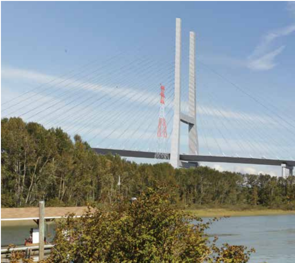
Rendering of the Overhead Transmission Line Alternative from Captain's Cove Marina, Delta (looking East-Northeast)
