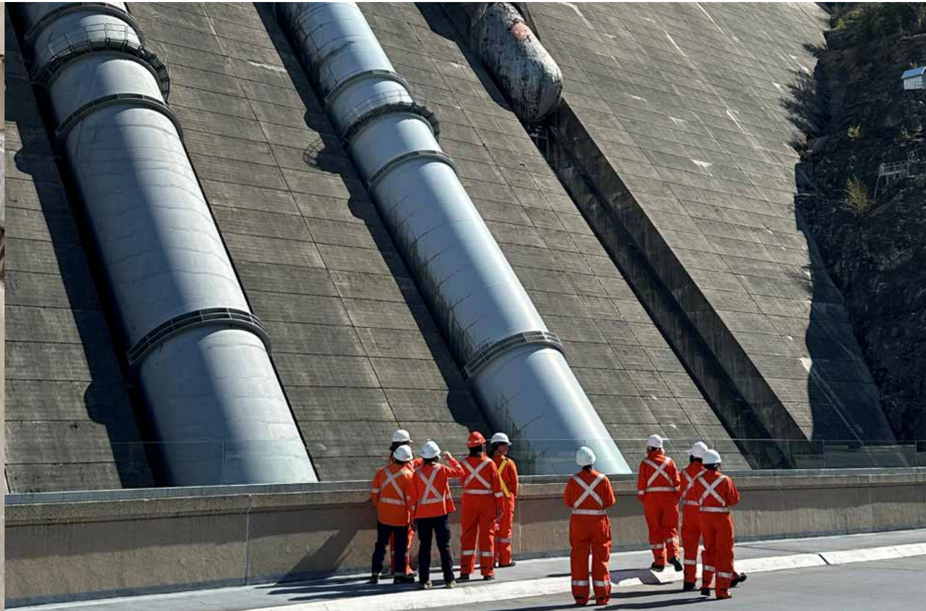
Space for new penstock
