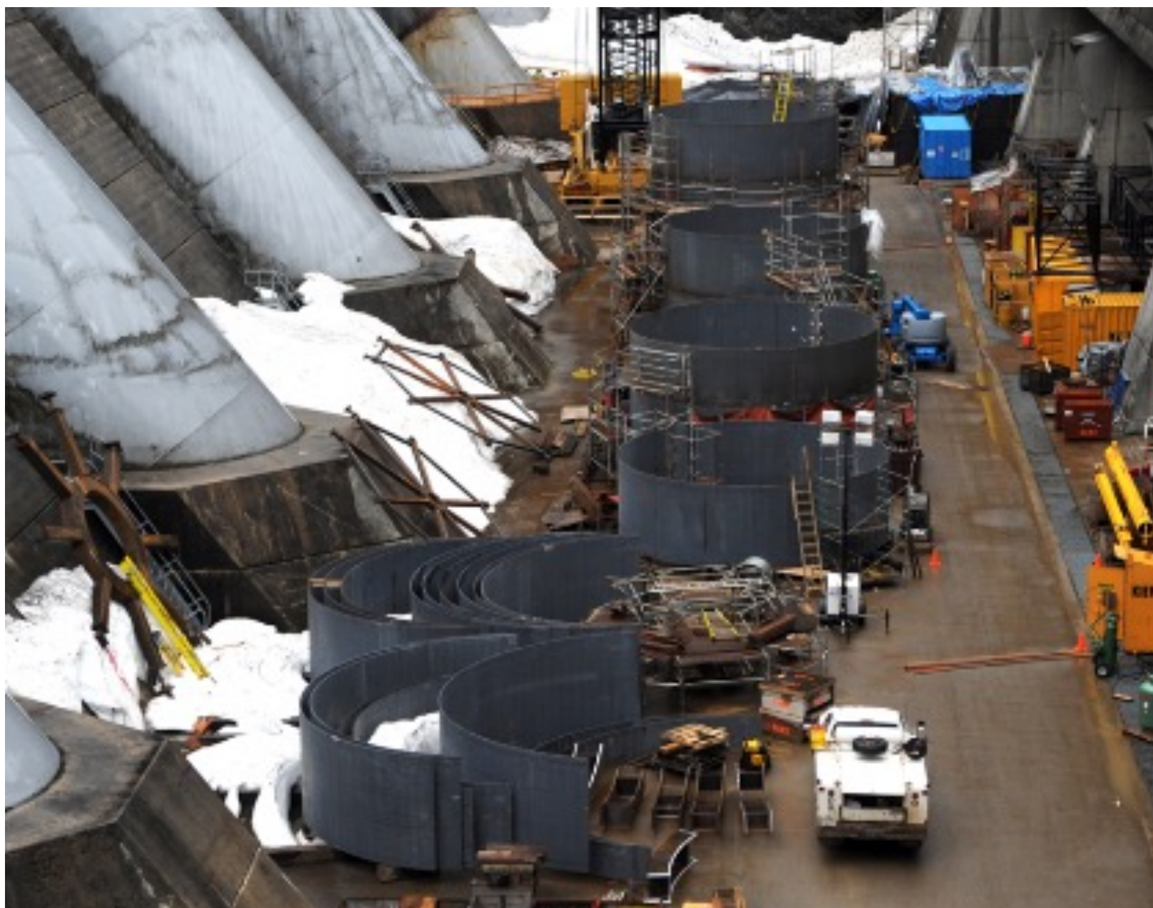
Rev 5 penstock work
