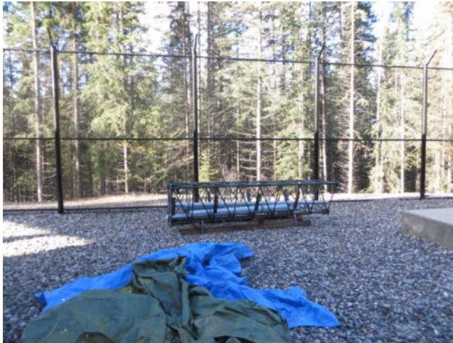
Figure 8 Satellite Tower to be erected
