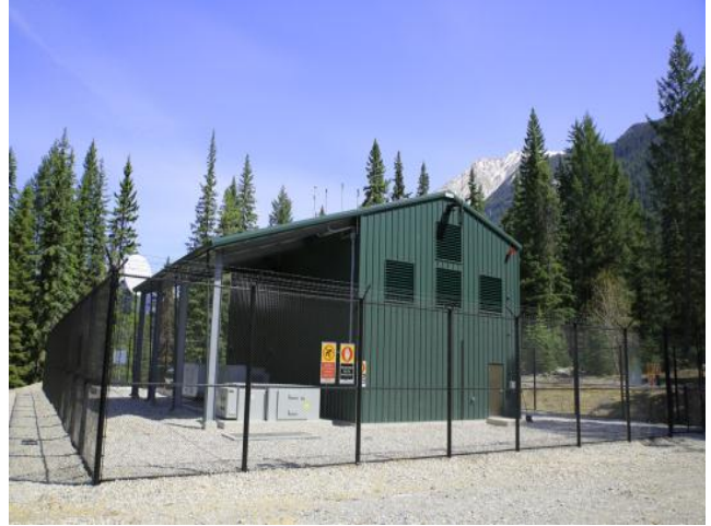
Figure 7 Completed Building facing North
