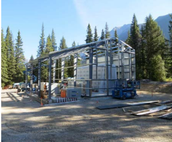
Figure 6 Structure being erected
