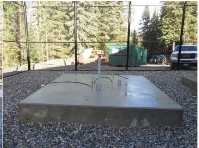
Figure 9 Socle de la tour satellite
