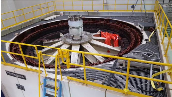
The Seton generating unit dismantled during annual maintenance.
