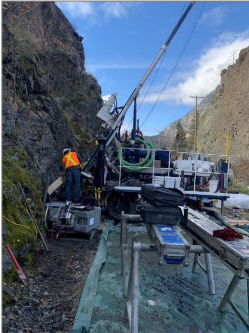
Crews drilling near the tie-in of the bypass and canal (Sept. 2021)
