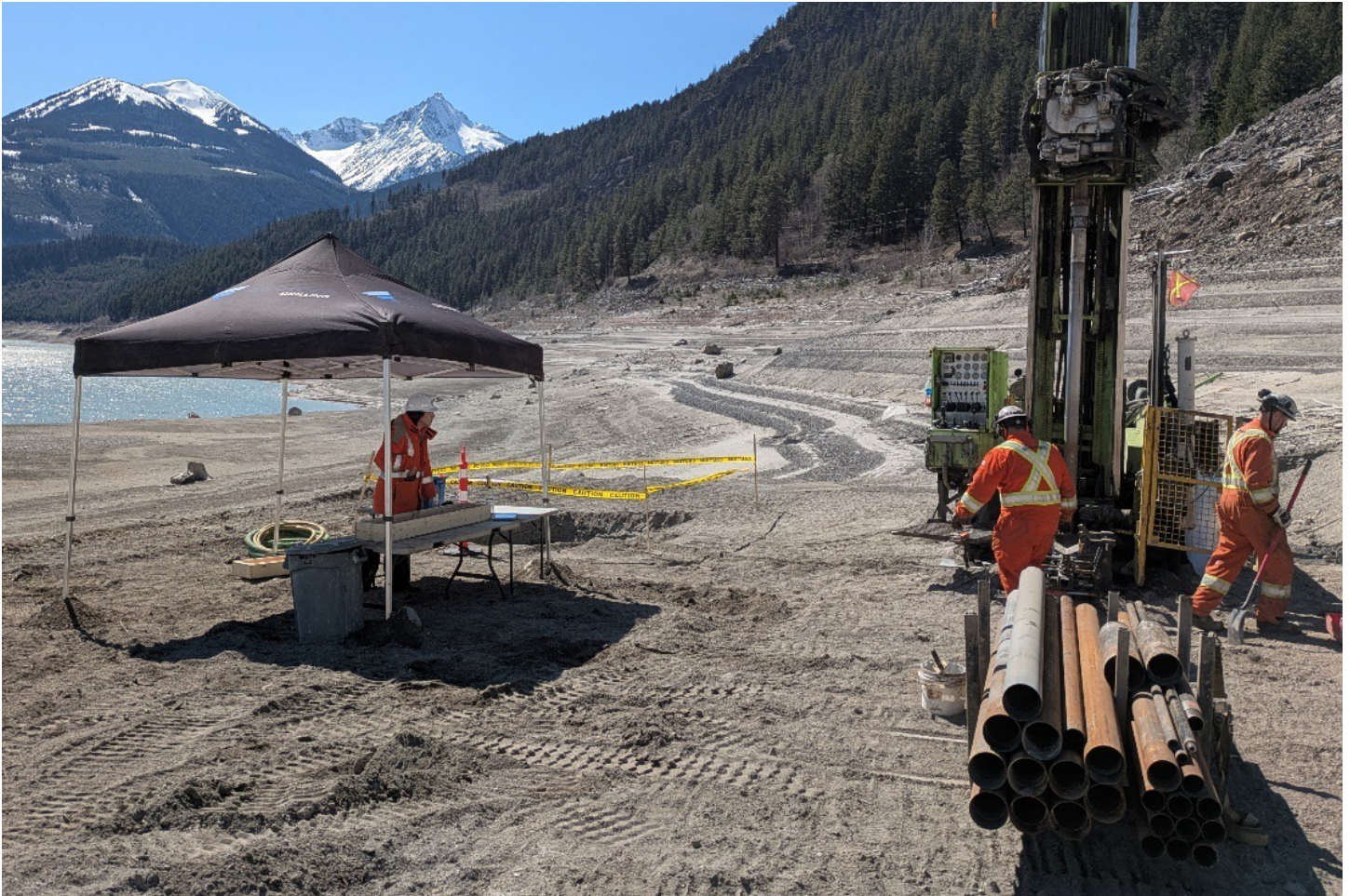
Crews working at La Joie Dam (April 2026)
