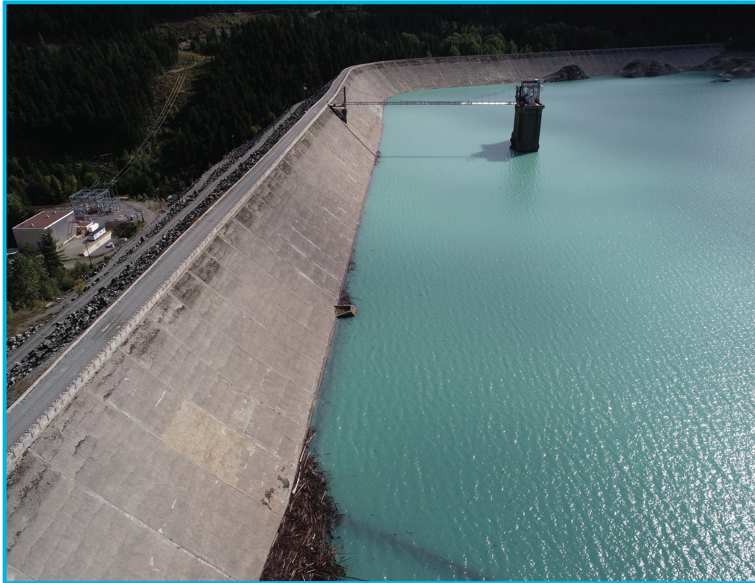
La Joie Dam and the intake tower standing in Downton Reservoir
