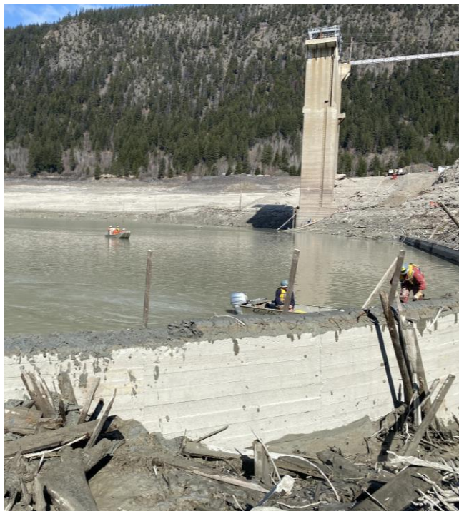
Crews investigating at the toe of the La Joie Dam during a drawdown (April 2022)
