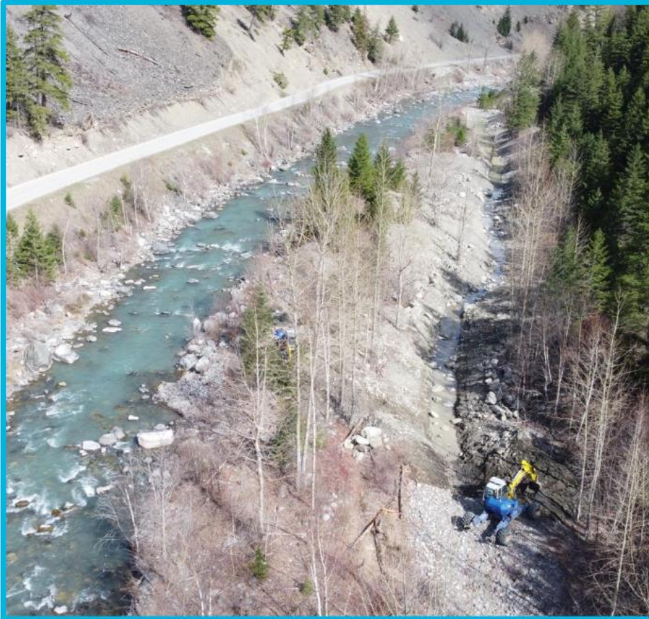
Grizzly Bar Side Channel during construction (March 2026)
