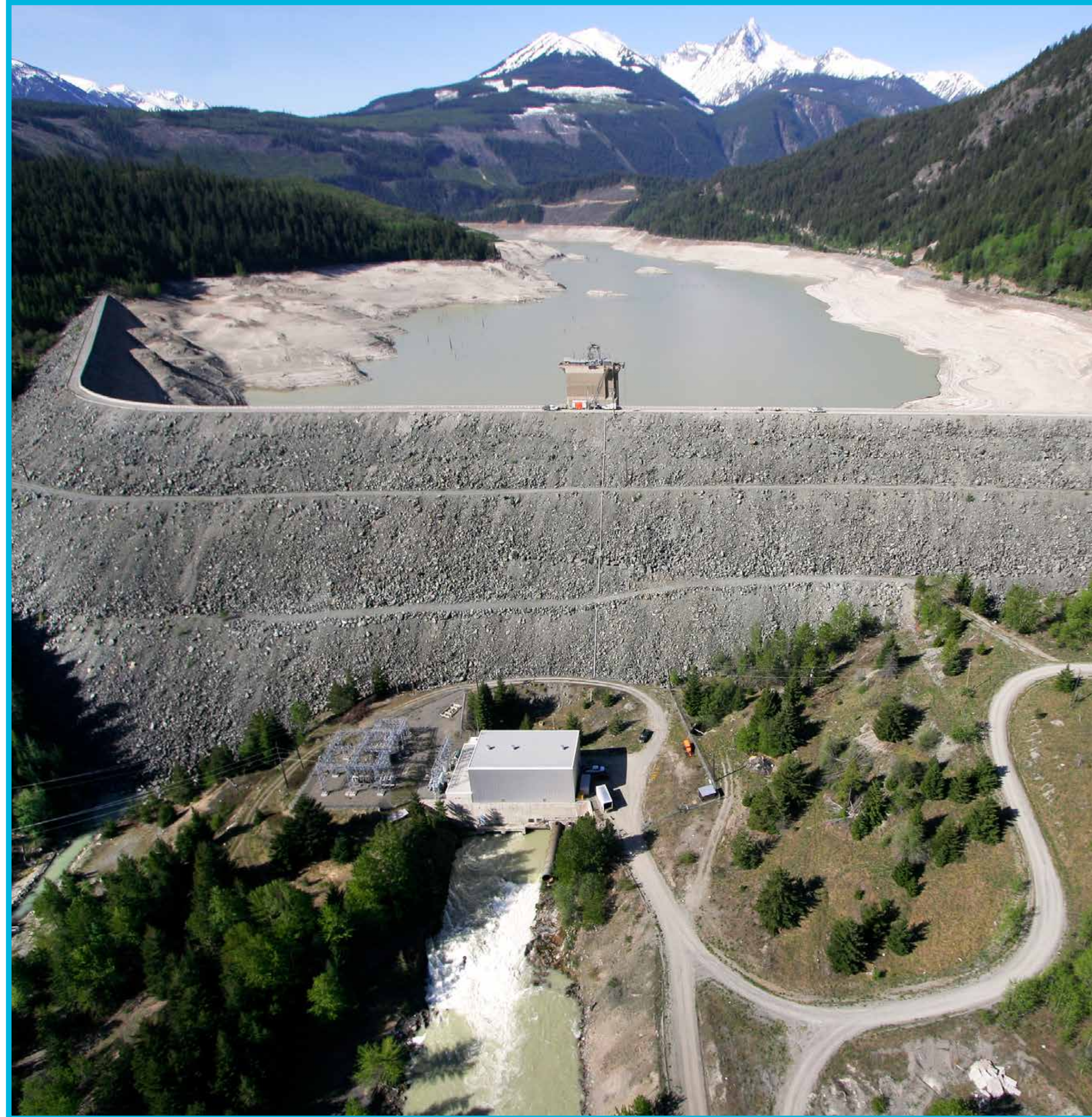
Aerial view of the La Joie Dam, powerhouse, and Downtown Reservoir.
