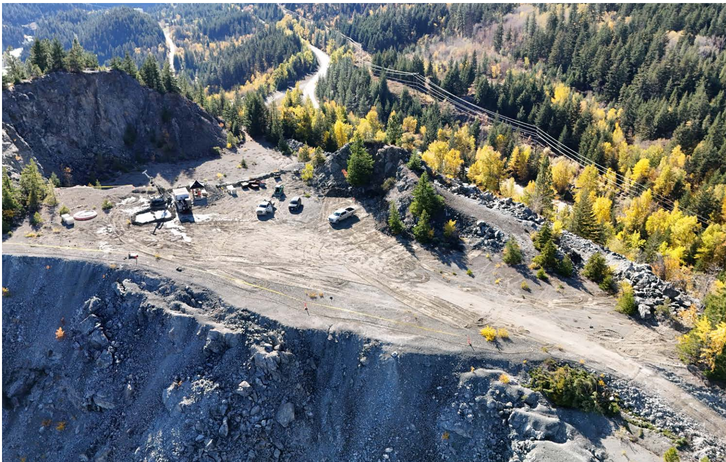
Crews conducting quarry investigations. (October 2025)
