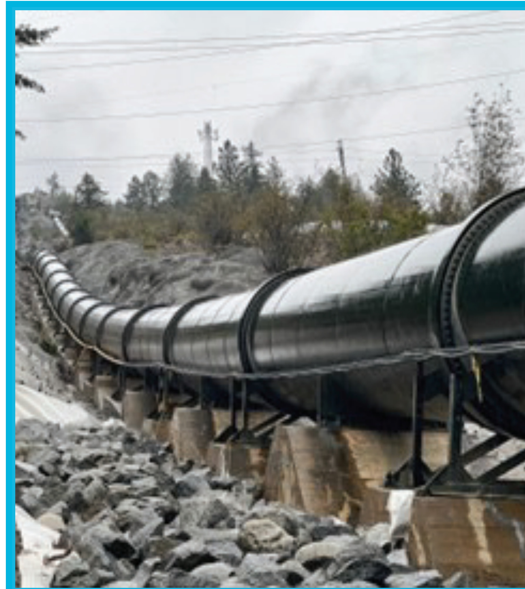
Exterior view of the Bridge 1 penstock
