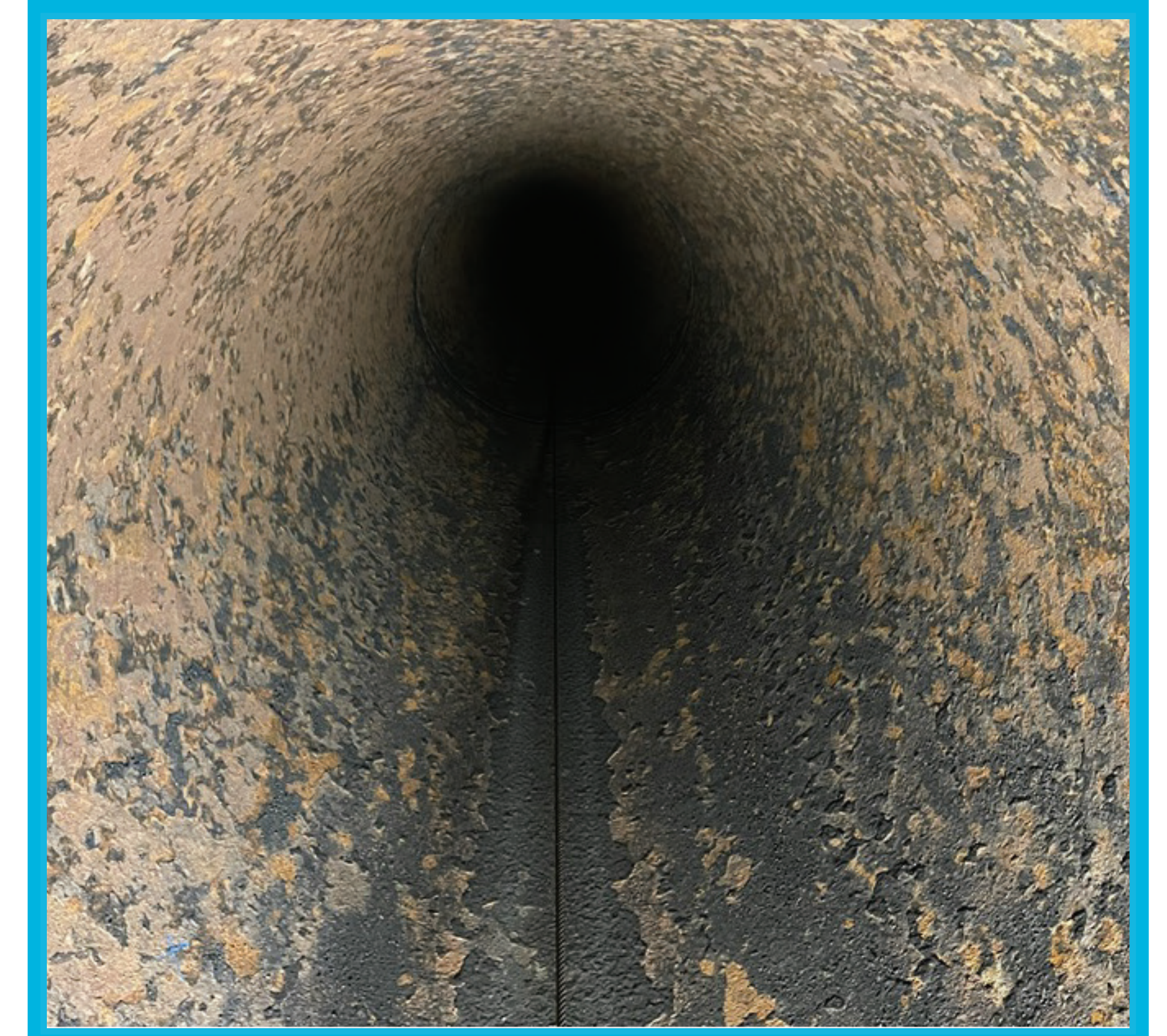
Inside the Bridge 1 penstock
